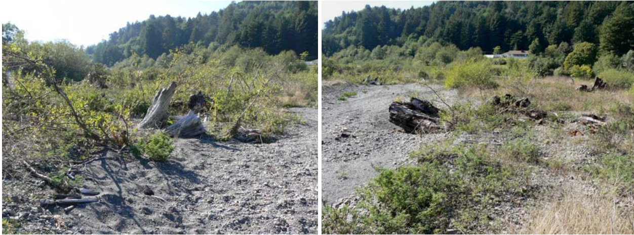
Figure 10. Photographs of large wood and willow planting islands installed in a constructed side channel feature of lower Terwer Creek.
