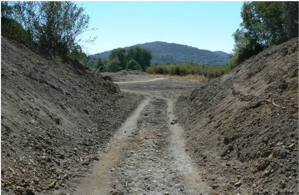
Figure 13. Photographs looking upstream at the breached levee and existing wetland habitats (Top) and looking downstream through the breached levee during off-channel habitat enhancement of Terwer Creek Pond B, Lower Klamath River (summer 2010).
