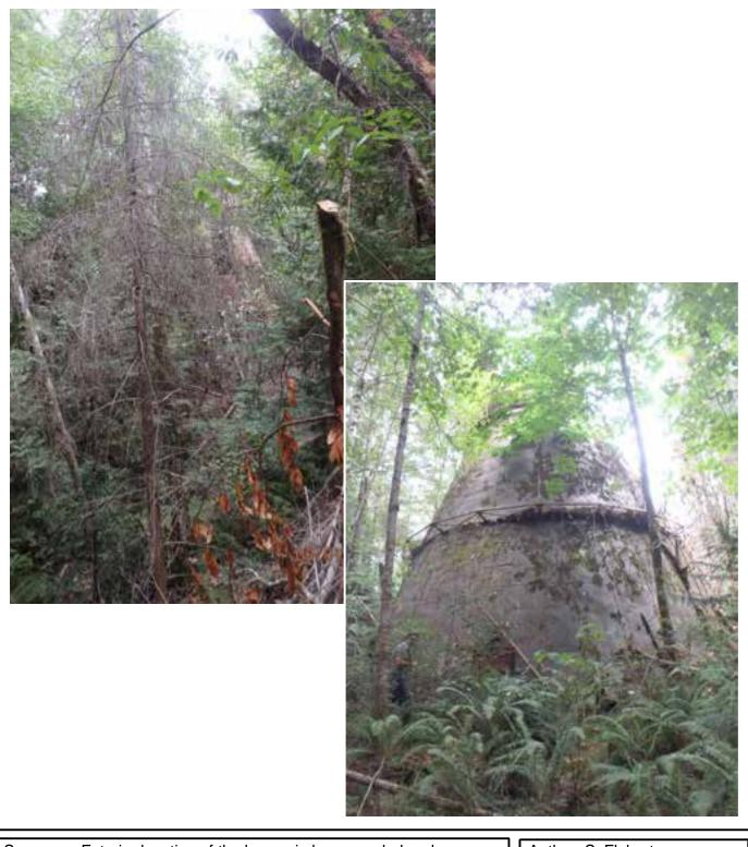
Summary: Exterior location of the burner in heavy underbrush. Upper Left: Looking downslope from the timber yard area. Lower Right: Looking upslope from dry water course used as access; Note ladder to right and inspection cat-walk half way up exterior wall. Author: S. Fluharty Date: September 1, 2016 APN: 534-091-18
