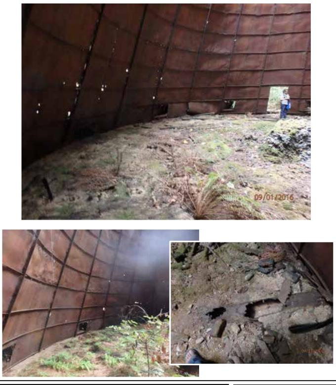
Summary: This shows the interior details of conical burner. Upper: Note the exposed ash pile and miscellaneous debris. Lower Left: Lower air vents & sparse vegetation compared to exterior. Lower Right: Corroded ignition pipe for burner.
