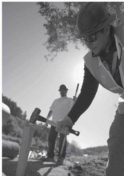
Thomas Marceau - Yurok Tribe Construction Corporation
