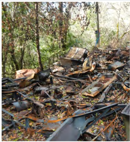
Many Tribal homes are trailers and burn extremely hot and quick, with an estimated 12-20 minutes total destruction time.
