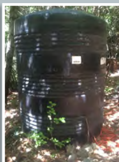
Typical water storage on gravity fed systems on the Yurok Reservation
