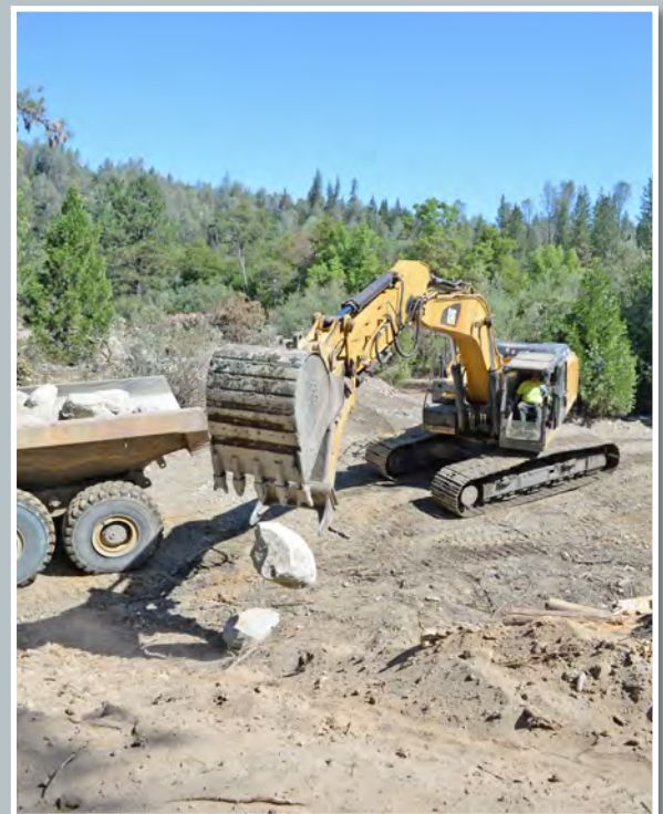
Yurok Watershed Restoration Department- working on logging road rehabilitation and stabilization
