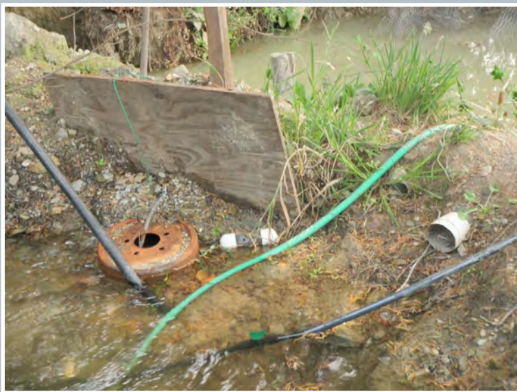
Private drinking water intake infrastructure on the Yurok Reservation is varied and often utilizes non-standard structures and piping
