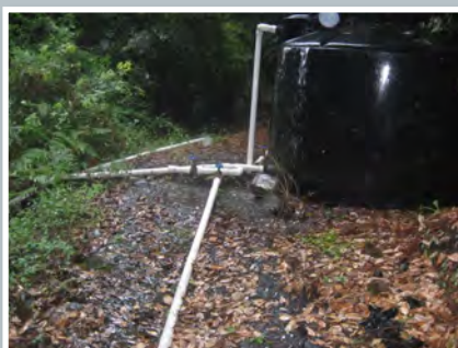
Typical water storage on gravity fed systems on the Yurok Reservation
