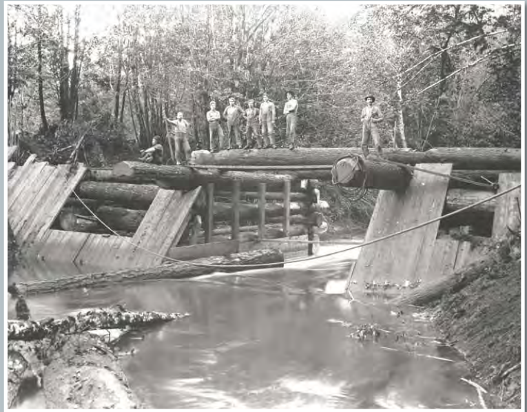
Example of a temporary 'splash' dam used in historic logging operations. Downloaded from: https://www.fs.fed.us/
