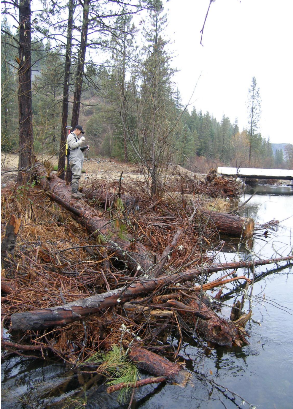
Figure 11. Slash incorporated into a large wood installation at Sawmill rehabilitation site. Large wood installations at previous sites did not incorporate slash, which increases the benefit of these installations to rearing salmonids. Slash increases the physical complexity of these features and therefore increases the quality of the escape-cover attributes for fish habitat.
