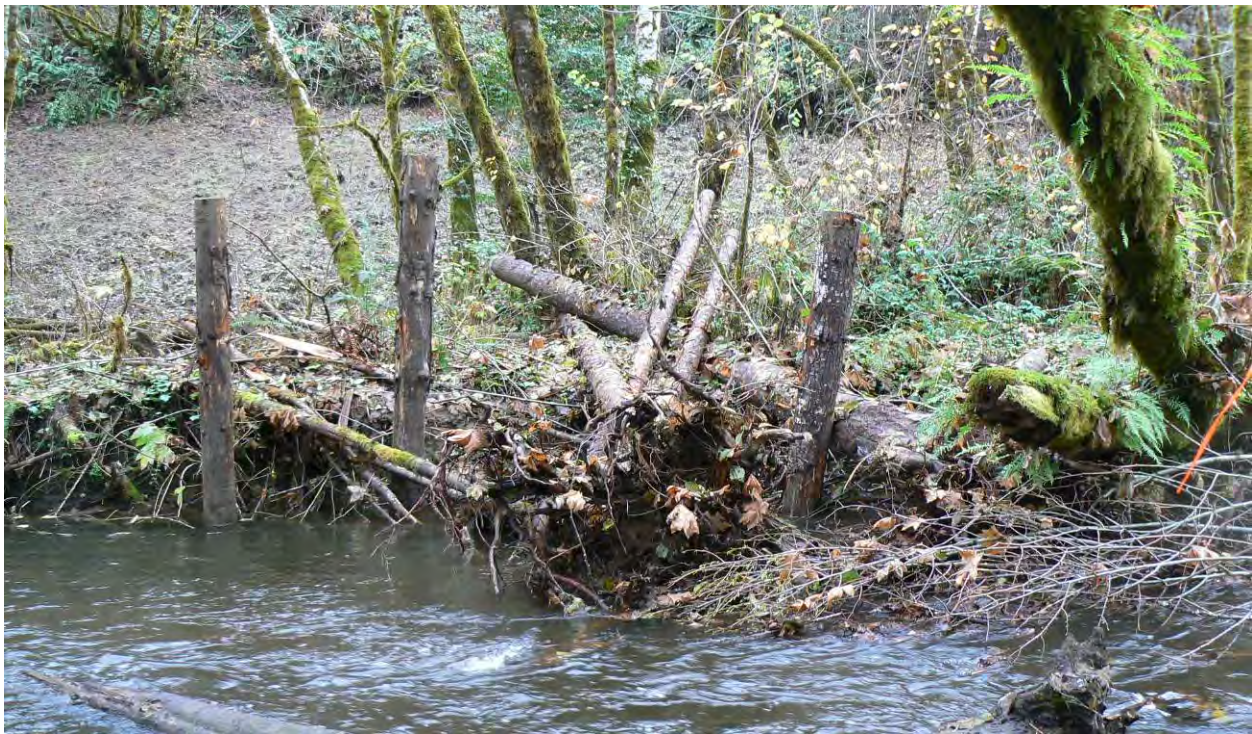
Photo-Site McG2013_E-1: Facing right bank towards 2013 CWJ Site 8 post-construction (11/20/13).
