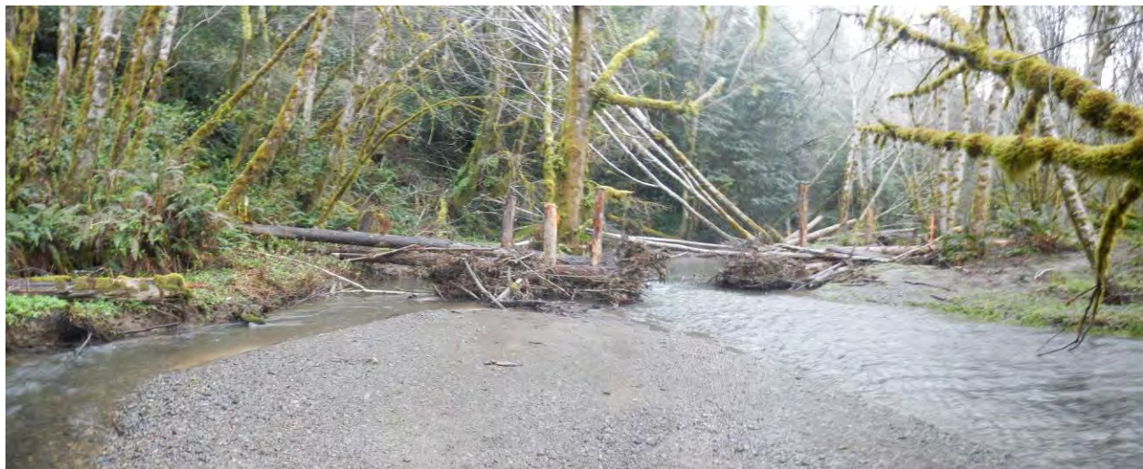
Figure 23. Looking downstream at constructed wood jams (McG_2013 Sites 4-5) installed in lower McGarvey Creek (02/26/14).
