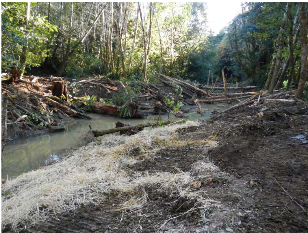
Figure 21. Looking upstream at McGarvey Alcove III during construction, 2013 (Top – alcove outlet prior to connecting the feature to McGarvey Creek; Bottom – alcove during excavation).
