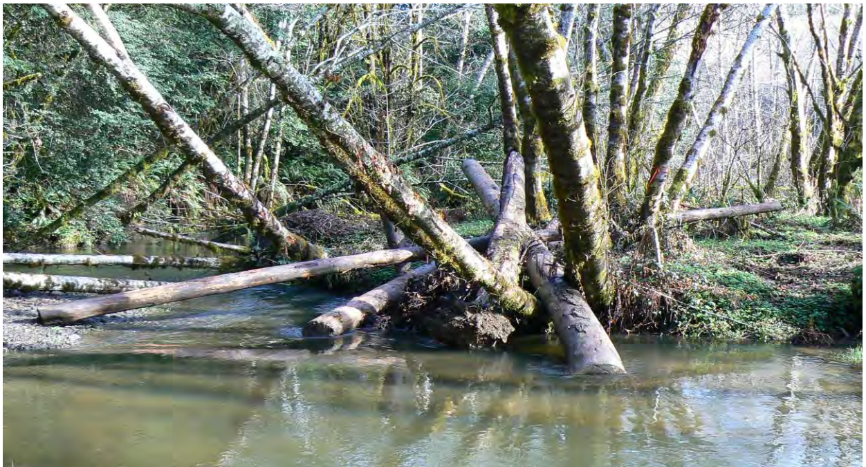
Photo-Site McG2013_C-1: 2013 CWJ Site 5 post-construction (02/10/14).
