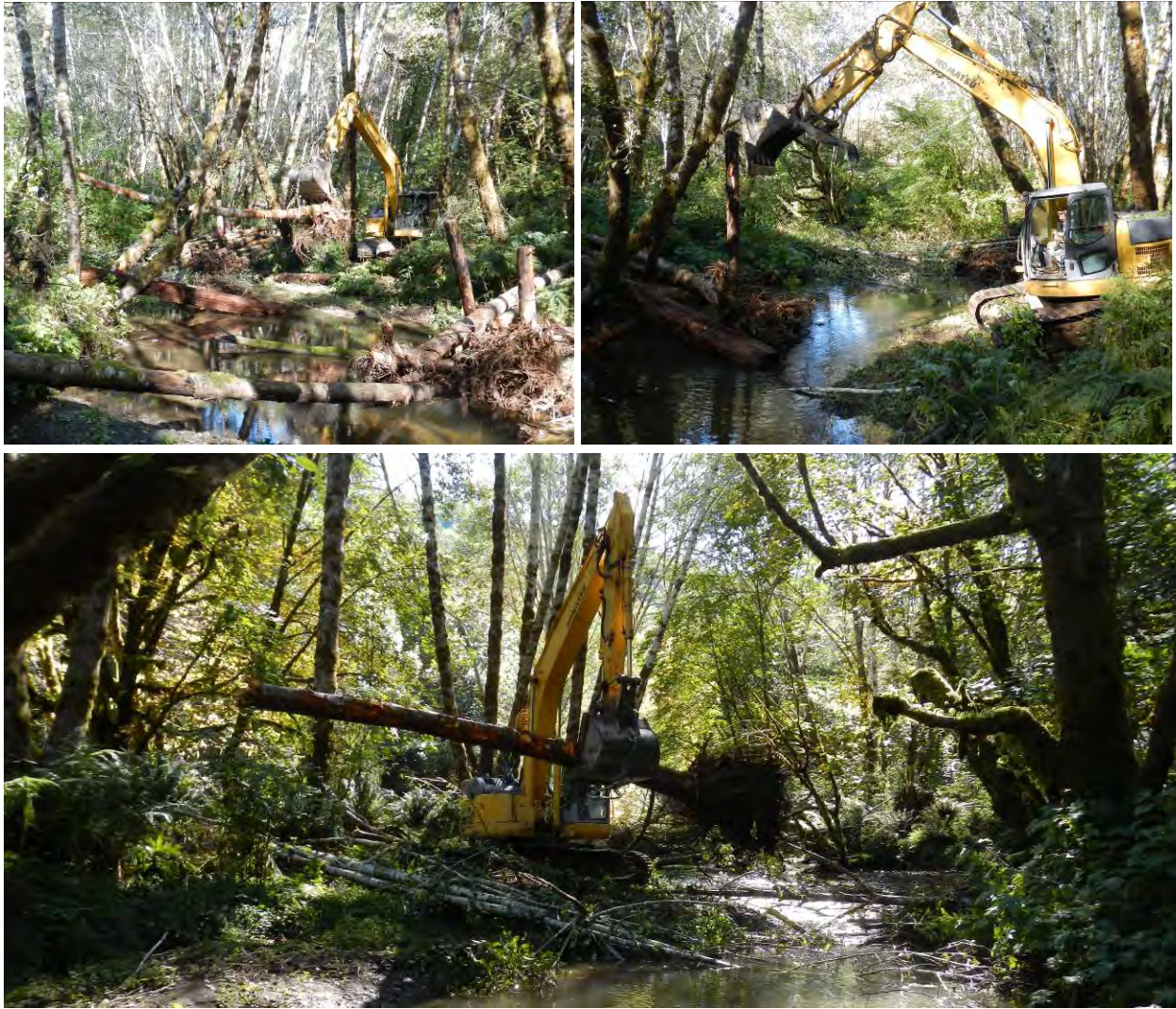
Figure 19. Rocco Fiori (Fiori GeoSciences) building constructed wood jams in McGarvey Creek, 2013 (Upper Left – Weaving a log with rootwad attached into riparian trees; Upper Right – setting a vertical pile for jam stability; Bottom – placing log with rootwad attached).
