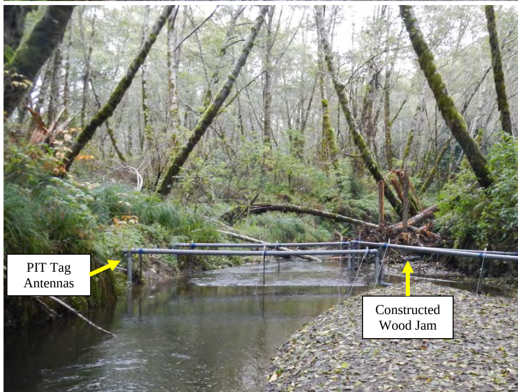
Figures 12. Photographs looking downstream at constructed wood jams installed in lower McGarvey Creek in summer 2012 (Photo Date: 11/13/12).
