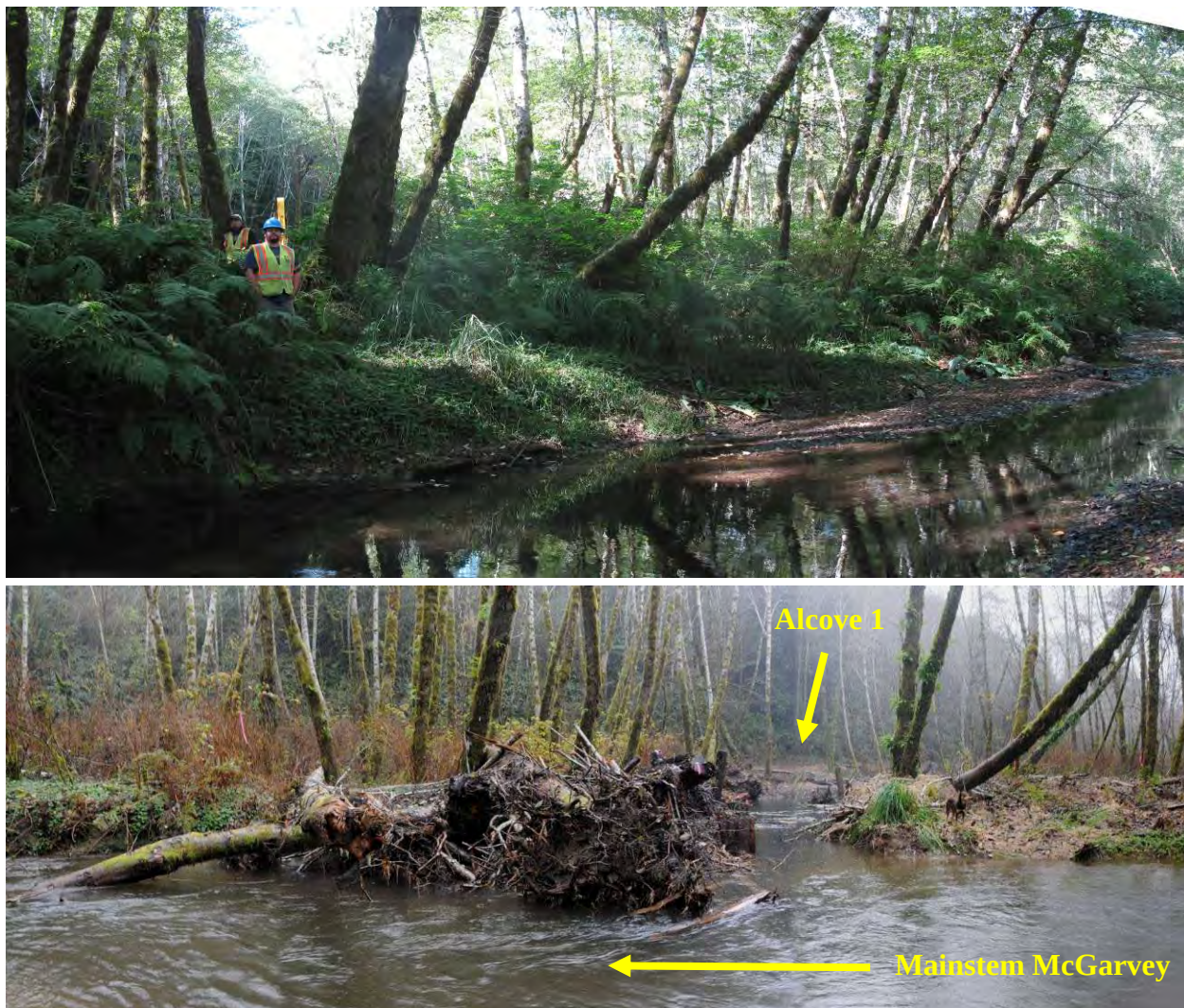
Figure 10. Photographs looking at the confluence of McGarvey Creek and Alcove I prior to construction (Top-2010) and during winter flows post-construction (Bottom-Winter 2011).
