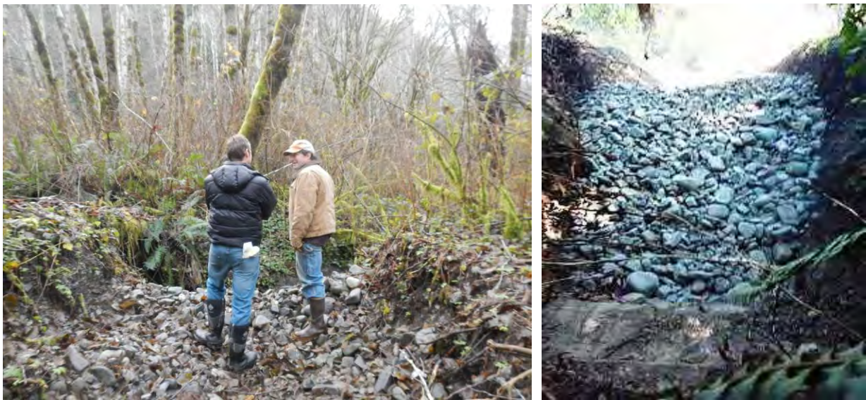
Figure 17. Photographs looking upstream at the rock sill during winter 2013 (Left) and the McGarvey Alcove II infiltration gallery channel post-construction in summer 2012 (Right).
