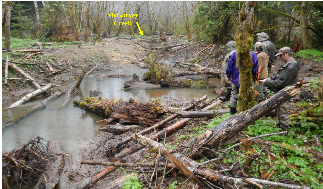
Figure 22. Looking downstream at McGarvey Alcove III post-construction (02/26/14).
