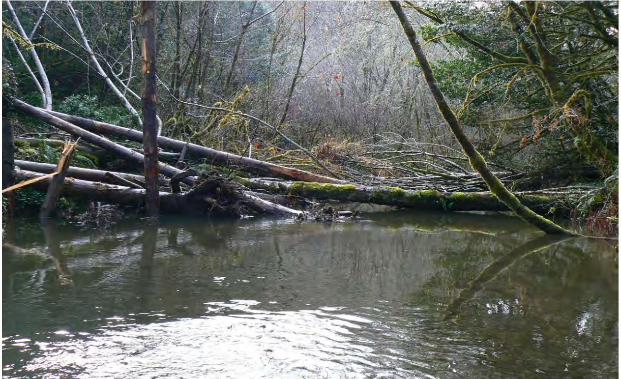
Photo-Site McG2013_A-1: Looking upstream at 2013 CWJ Site 1 post-construction (02/10/14).
