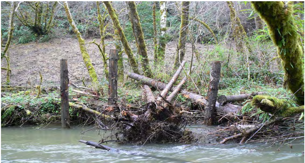
Photo-Site McG2013_E-1: 2013 CWJ Site 8 post-construction (02/19/14).
