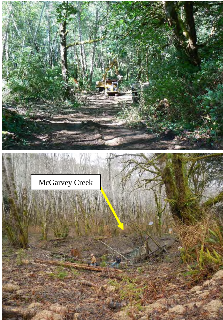
Figure 14. Photographs looking downstream at McGarvey Creek Alcove II prior to construction (Top-09/10/12) and during winter flows post-construction (Right-01/03/13).
