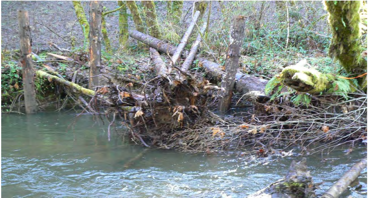
Photo-Site McG2013_E-1: 2013 CWJ Site 8 post-construction (02/10/14).
