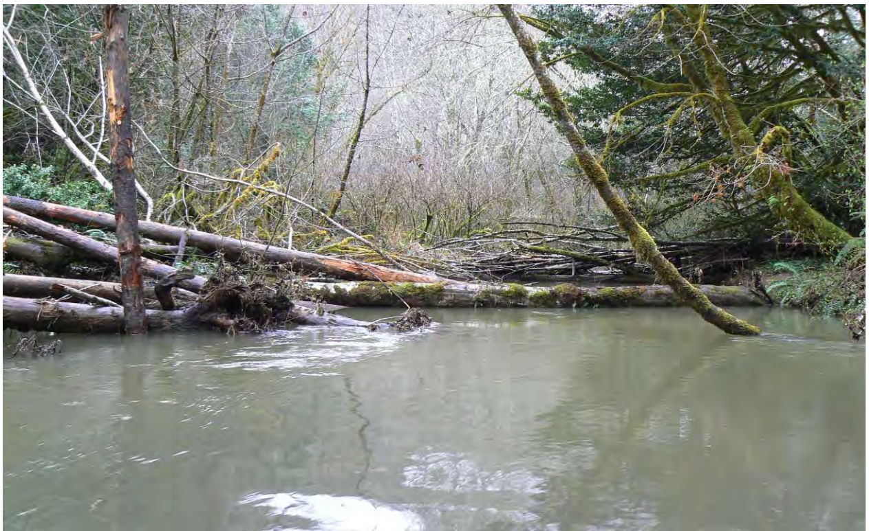
Photo-Site McG2013_A-1: Looking upstream at 2013 CWJ Site 1 post-construction (02/19/14).
