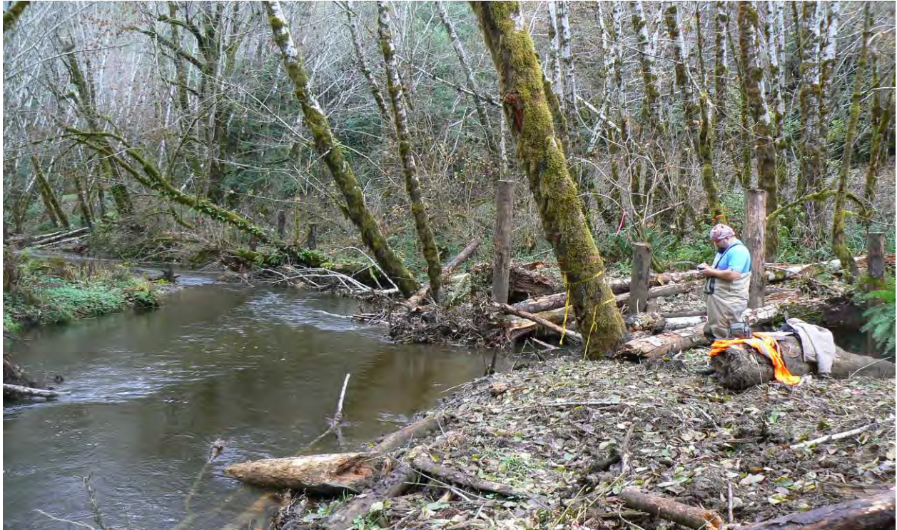
Photo-Site McG2013_D-2: Looking downstream at 2013 CWJ Site 7 post-construction (11/20/13).
