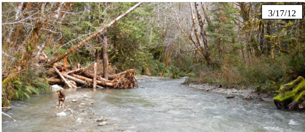
Figure 3. Constructed wood jam in East Fork Hunter Creek in the first spring post-construction.
