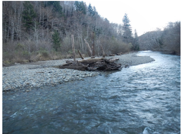
Figure 5. A bar apex jam (USFWS Site 2) during construction (Top, Middle – Aug. 2012) and during the first winter-spring post-construction (Bottom Left 11/20/12 – Bottom Right 3/7/13).
