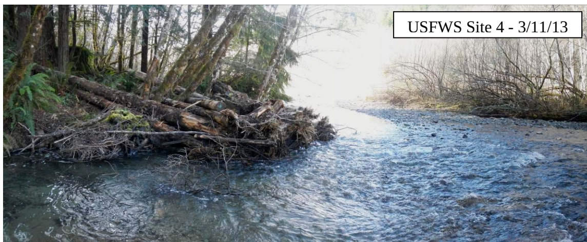
Figure 4. Constructed wood jam in Hunter Creek in the first spring post-construction.
