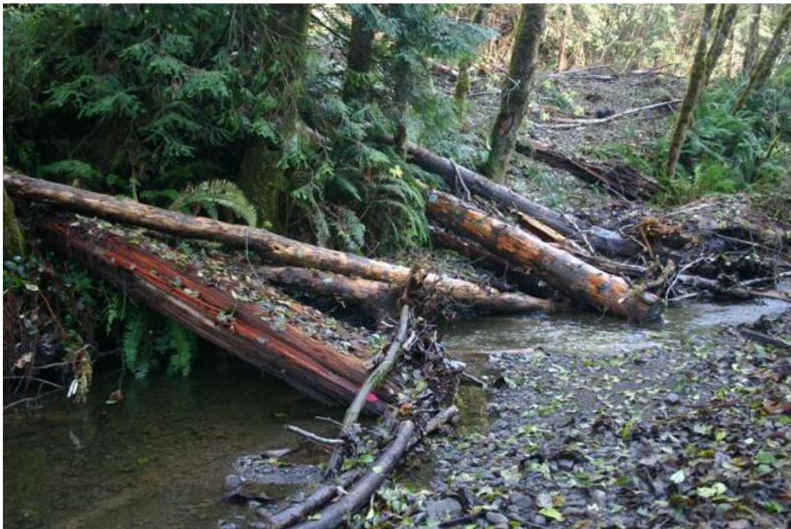
Figure 101. Scour pool habitat following installation of structure #15, Mainstem McGarvey Creek, Lower Klamath River, California, November 2008.
