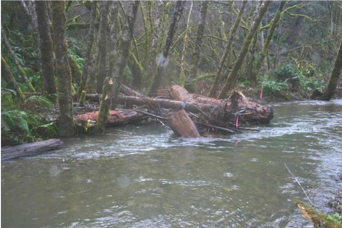
Figure 108. Structure #17 following high winter flows, Mainstem McGarvey Creek, Lower Klamath River, California, January 2009.
