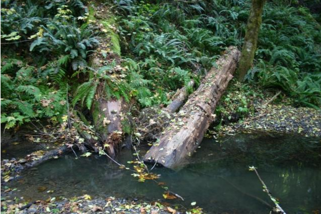
Figure 84. Scour pool in middle portion of reach following installation of structure #12, Mainstem McGarvey Creek, Lower Klamath River, California, October 2008.
