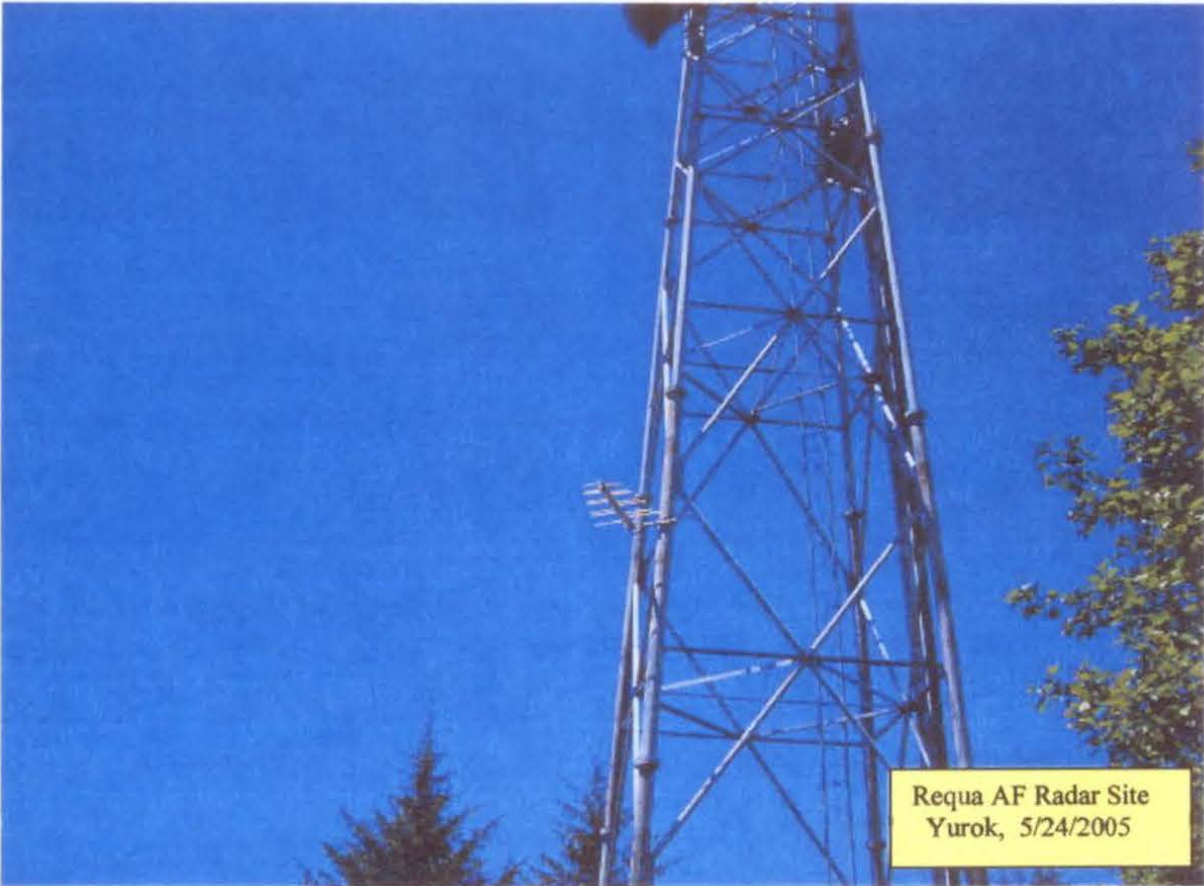
Standing on the concrete radar pad and looking Southwest at the adjacent property at the cell phone tower presently in operation.
