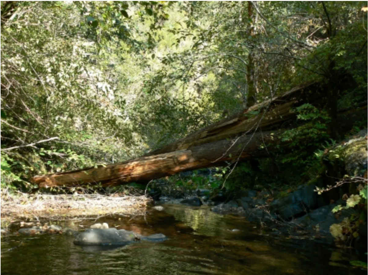
Figure 12. Photographs of Douglas fir cull logs flown and placed in the lower seven miles of Tectah Creek, Lower Klamath River Sub-basin, California (September - October 2008).
