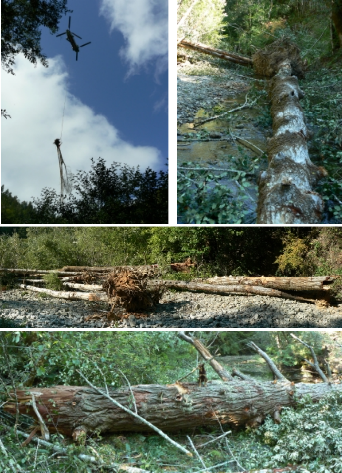
Figure 11. Photographs of tan oak that were flown and placed in the lower seven miles of Tectah Creek, Lower Klamath River Sub-basin, California (September 2008).
