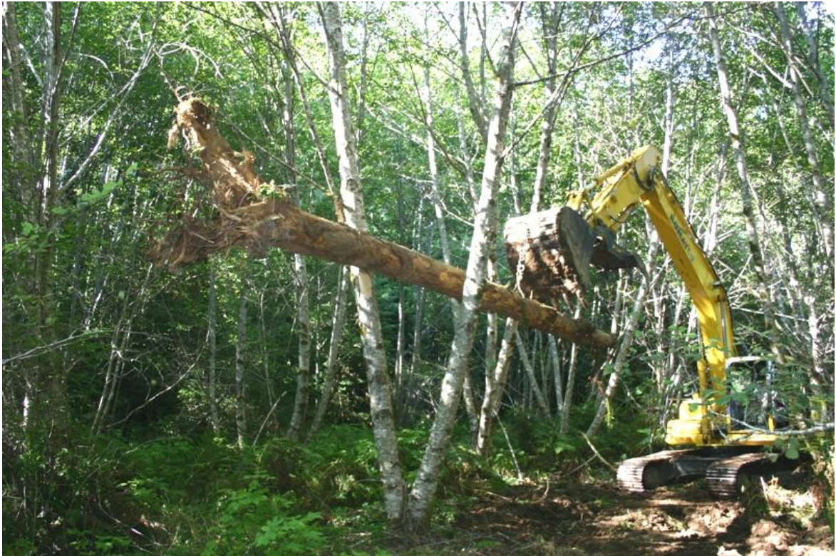
Figure 19. Positioning LWD between anchor trees along stream channel, West Fork McGarvey Creek, Lower Klamath River, California, 2007.
