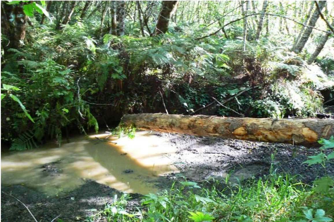
Figure 21. Fir log being plunged into streambank with excavator, West Fork McGarvey Creek, Lower Klamath River, California, 2007.
