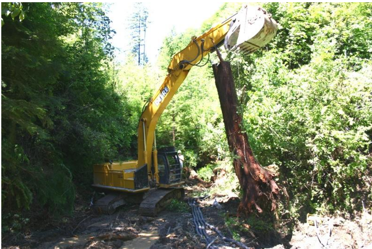
Figure 13. Large woody debris retrieved from “Humboldt” stream crossing during road decommissioning, McGarvey Creek, Lower Klamath River, California 2006.
