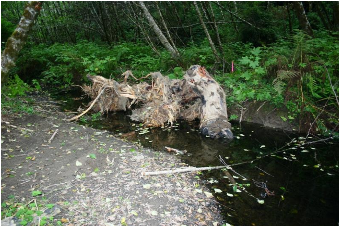
Figure 54. Shallow pool following installation of LWD pieces #22-26, West Fork McGarvey Creek, Lower Klamath River, California, 2007.
