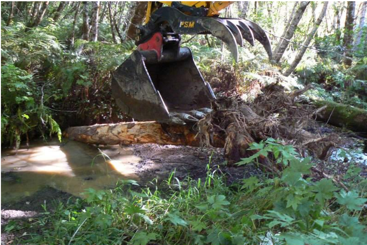
Figure 23. Fir log being plunged into streambank with excavator, West Fork McGarvey Creek, Lower Klamath River, California, 2007.
