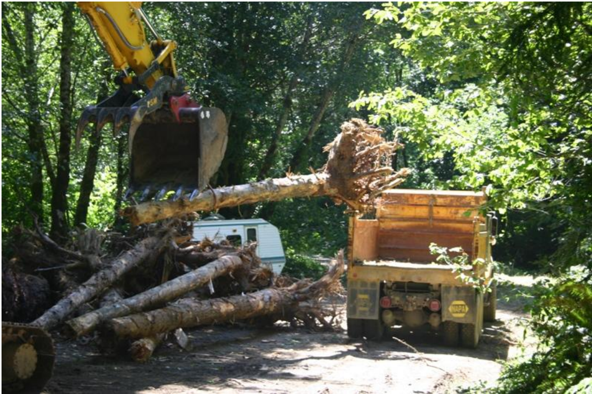
Figure 15. Road decommissioning-salvaged LWD being unloaded at West Fork stockpile area, McGarvey Creek, Lower Klamath River, California, 2007.
