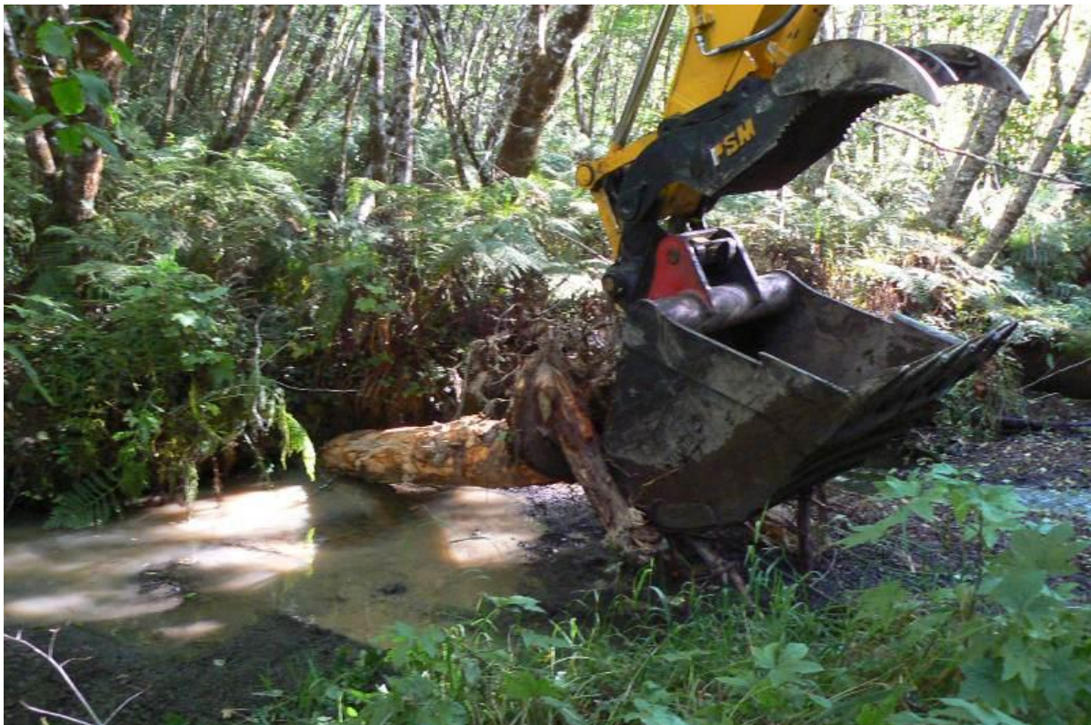
Figure 24. Fir log being plunged into streambank with excavator, West Fork McGarvey Creek, Lower Klamath River, California, 2007.
