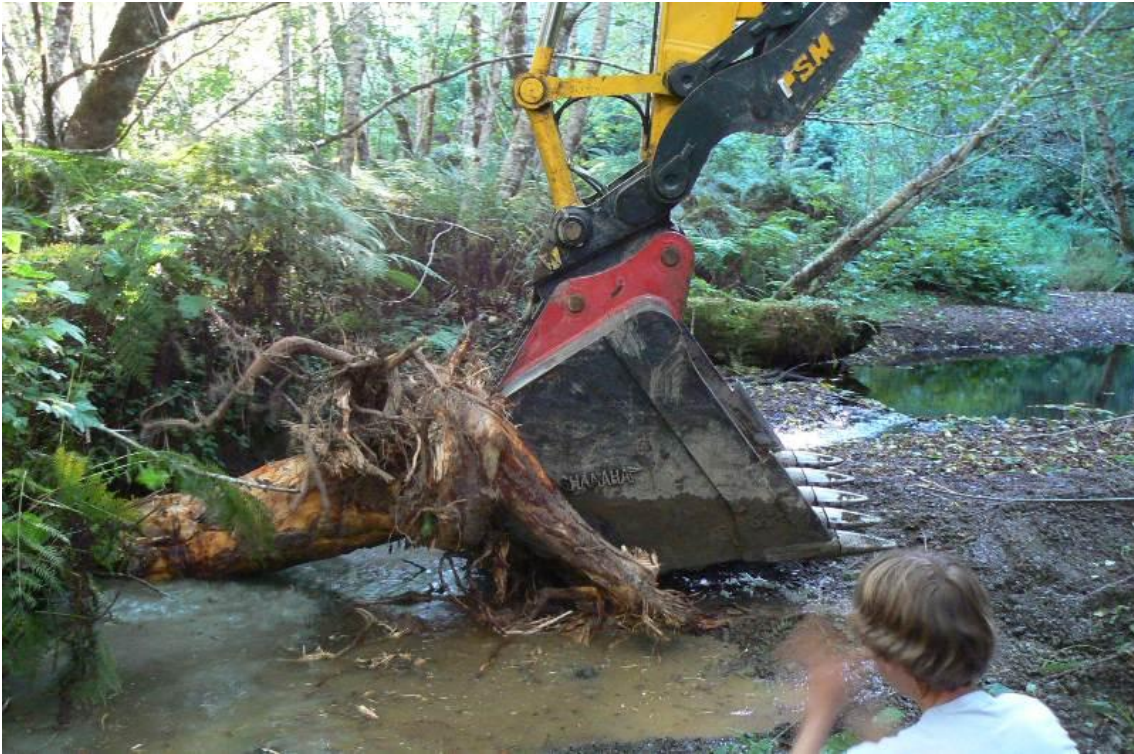
Figure 25. Fir log being plunged into streambank with excavator, West Fork McGarvey Creek, Lower Klamath River, California, 2007.
