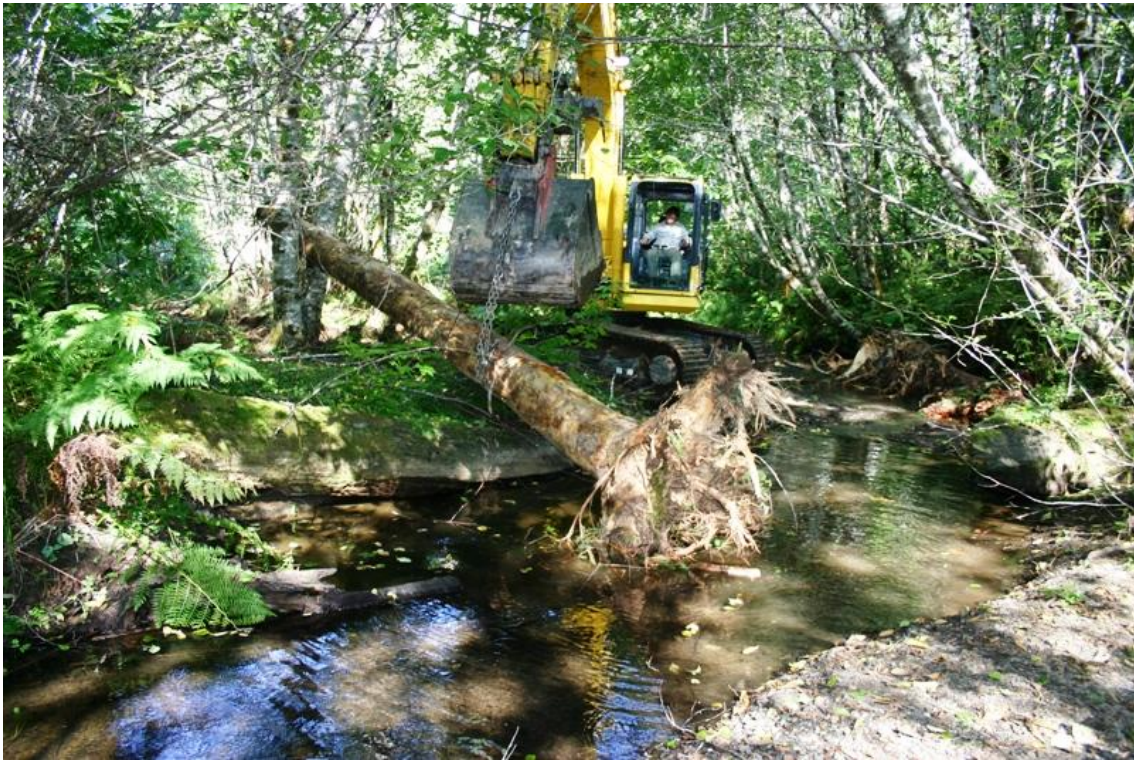
Figure 29. Shallow pool near top end of project reach during installation of LWD pieces #2-4, West Fork McGarvey Creek, Lower Klamath River, California, 2007.
