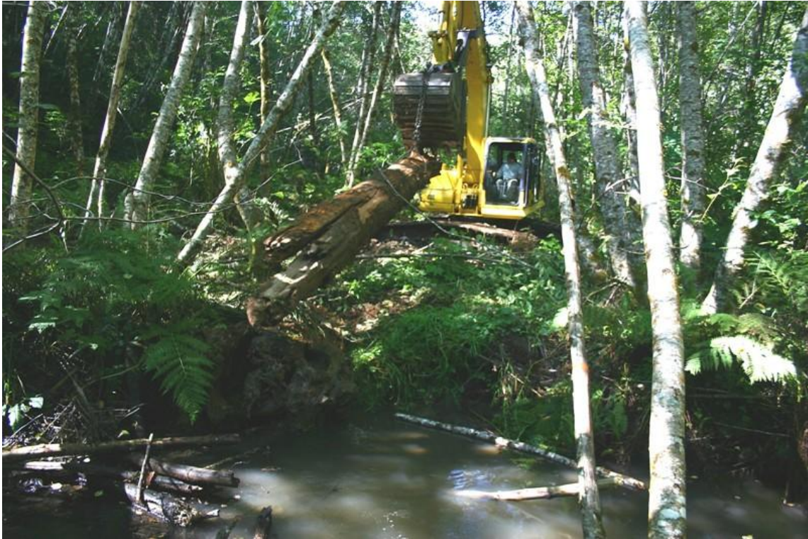
Figure 47. Shallow pool during installation of LWD pieces #18-21, West Fork McGarvey Creek, Lower Klamath River, California, 2007.
