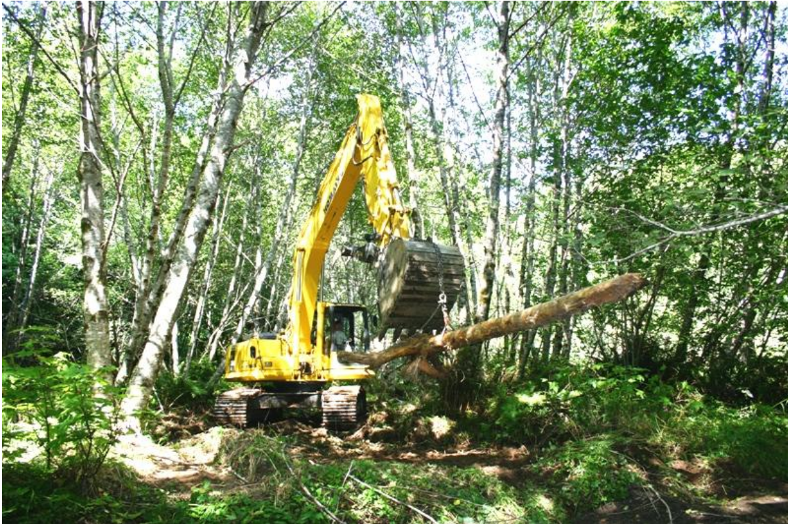
Figure 17. Transporting LWD to stream channel, West Fork McGarvey Creek, Lower Klamath River, California, 2007.
