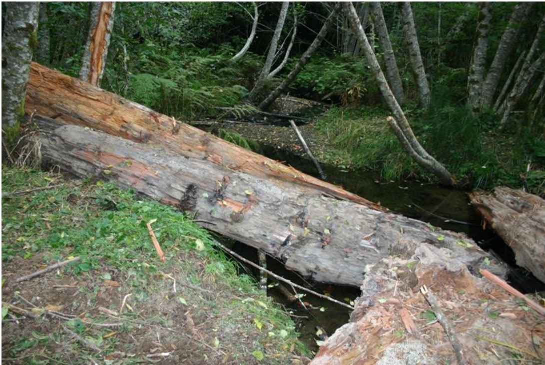
Figure 64. Shallow pool following installation of LWD pieces #31-34, West Fork McGarvey Creek, Lower Klamath River, California, 2007.
