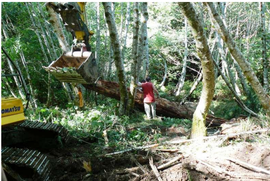
Figure 62. Shallow pool during installation of LWD pieces #31-34, West Fork McGarvey Creek, Lower Klamath River, California, 2007.
