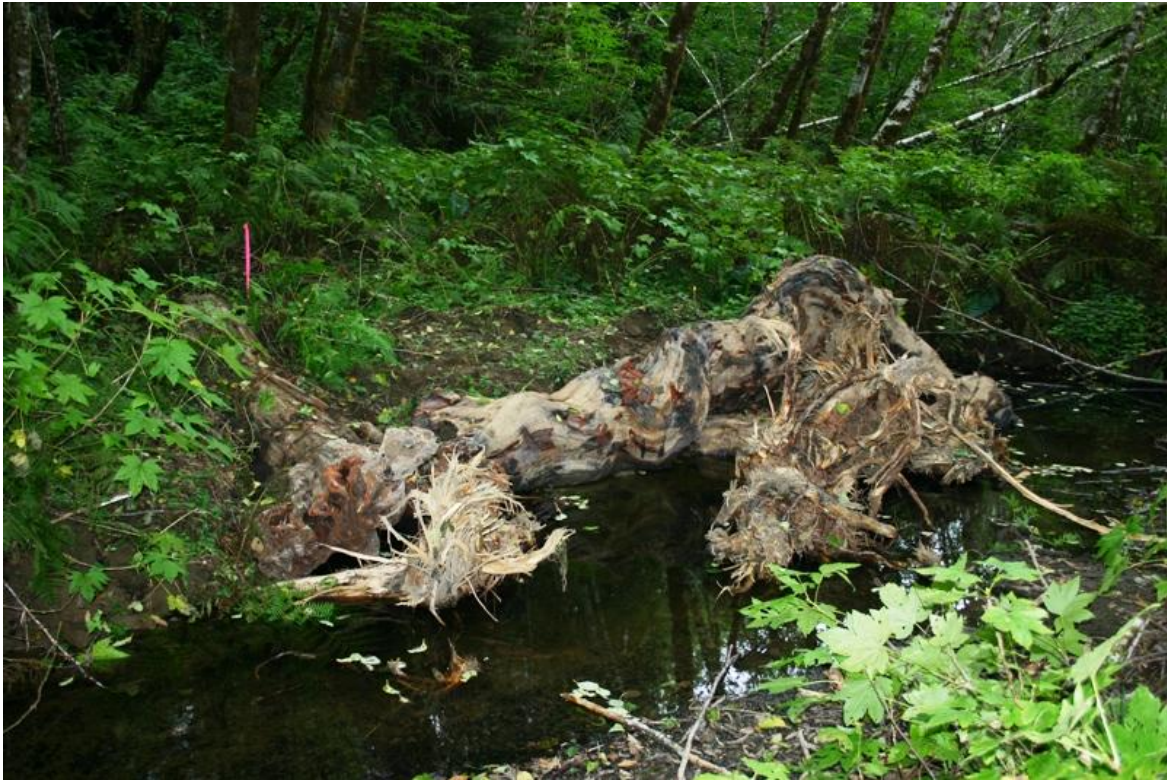
Figure 55. Shallow pool following installation of LWD pieces #22-26, West Fork McGarvey Creek, Lower Klamath River, California, 2007.
