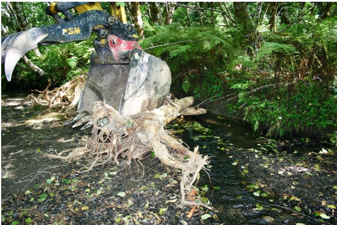
Figure 34. Shallow pool near top of project reach during installation of LWD pieces #5-10, West Fork McGarvey Creek, Lower Klamath River, California, 2007.
