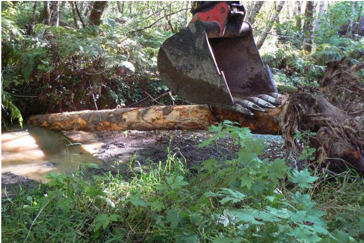
Figure 22. Fir log being plunged into streambank with excavator, West Fork McGarvey Creek, Lower Klamath River, California, 2007.
