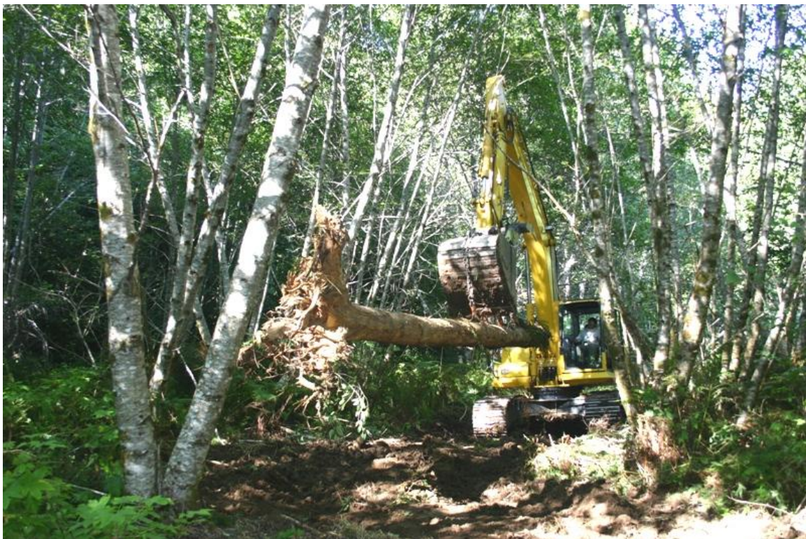
Figure 18. Transporting LWD to stream channel, West Fork McGarvey Creek, Lower Klamath River, California, 2007.
