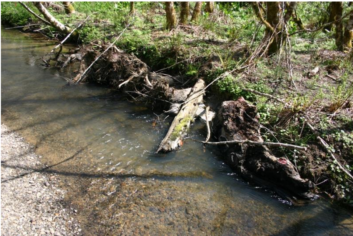
Figure 36. LWD pieces #5-10 following first winter, West Fork McGarvey Creek, Lower Klamath River, California, 2008.
