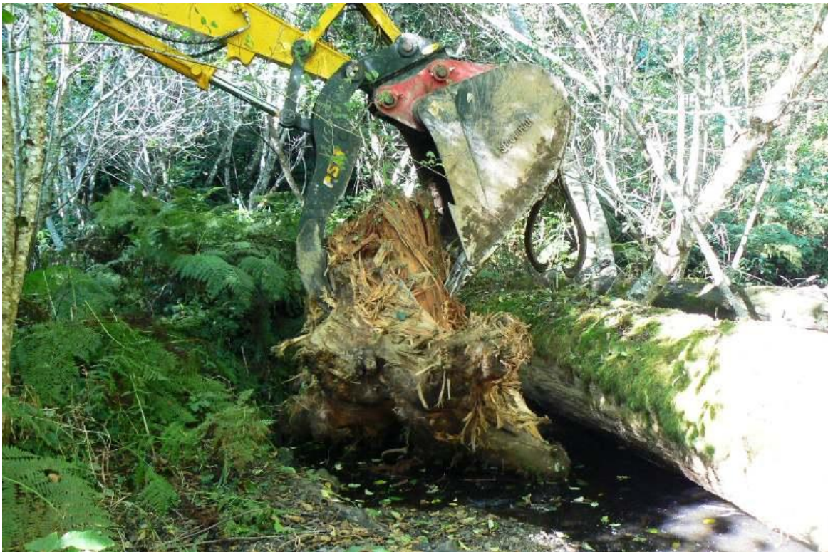
Figure 42. Rootwad (LWD piece #17) being placed in backwater pool, West Fork McGarvey Creek, Lower Klamath River, California, 2007.
