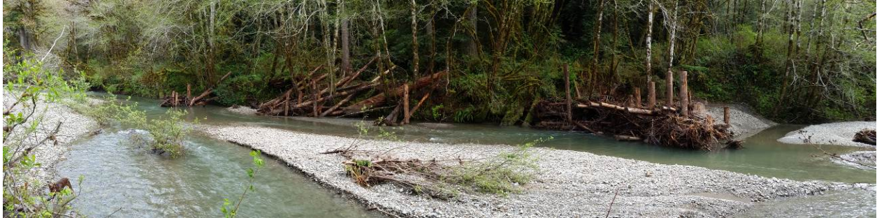
Figure 3. Constructed wood jams in Hunter Creek during a high flow event (03/20/16).
