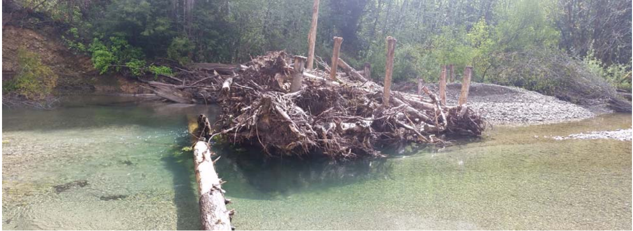
Figure 4. A constructed wood jam (Chaos Jam) in Hunter Creek (04/04/16).
