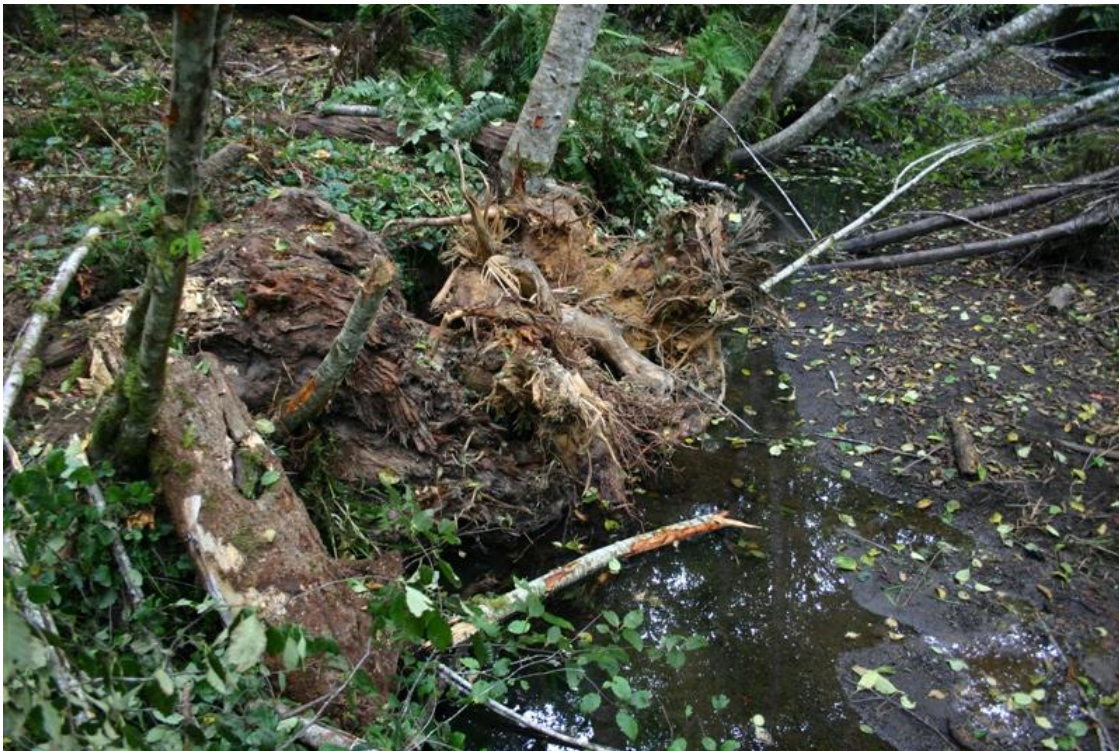
Figure 73. Shallow pool following installation of LWD pieces #35-41, West Fork McGarvey Creek, Lower Klamath River, California, 2007.
