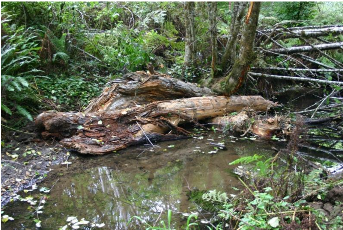
Figure 77. Shallow pool in lower end of project reach after installation of LWD pieces #42-45, West Fork McGarvey Creek, Lower Klamath River, California, 2007.
