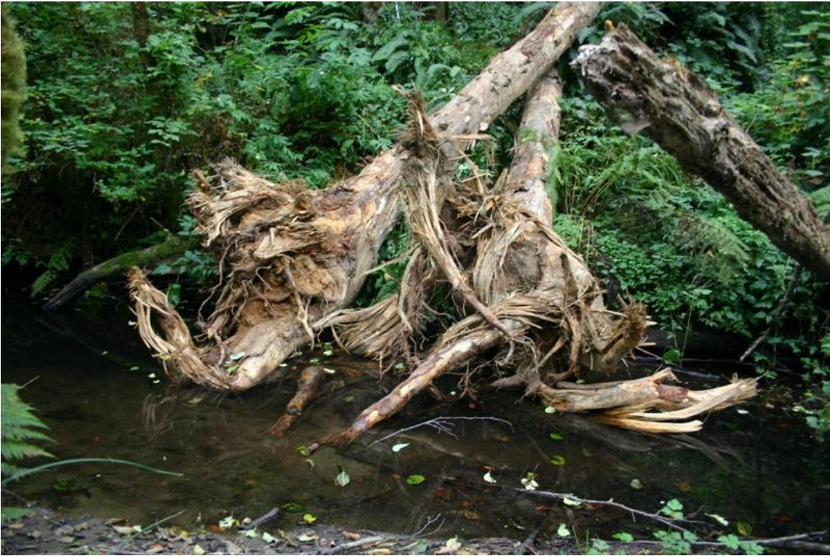
Figure 87. Shallow pool in lower end of project reach after installation of LWD pieces #48-49, West Fork McGarvey Creek, Lower Klamath River, California, 2007.
