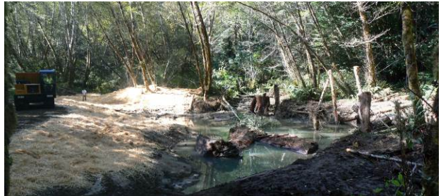
Figure 8. Placement of erosion control hay at McGarvey Creek Alcove IV following construction (Left – Looking downstream 10/13/14; Right – Looking upstream 10/13/14).
