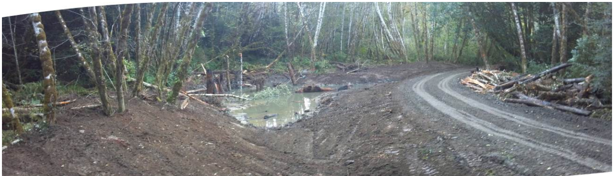
Photo-Site McGAlcoveIV_1: McGarvey Creek Alcove IV during construction (10/13/2014).
