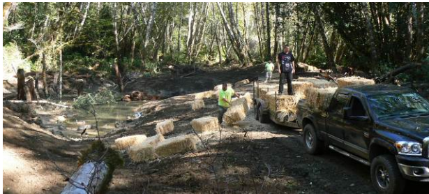
Figure 8. Placement of erosion control hay at McGarvey Creek Alcove IV following construction (Left – Looking downstream 10/13/14; Right – Looking upstream 10/13/14).
