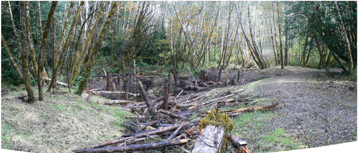
Photo-Site McGAlcoveIV_1: McGarvey Creek Alcove IV post-construction (10/31/2014).
