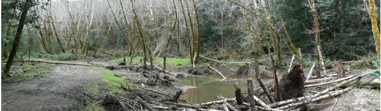
Figure 10. McGarvey Creek Alcove IV during the first winter post-construction (02/12/15).
