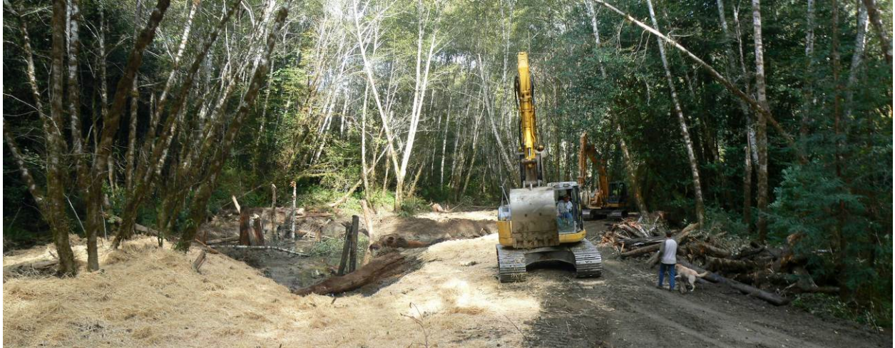
Photo-Site McGAlcoveIV_1: McGarvey Creek Alcove IV during construction (10/14/2014).
