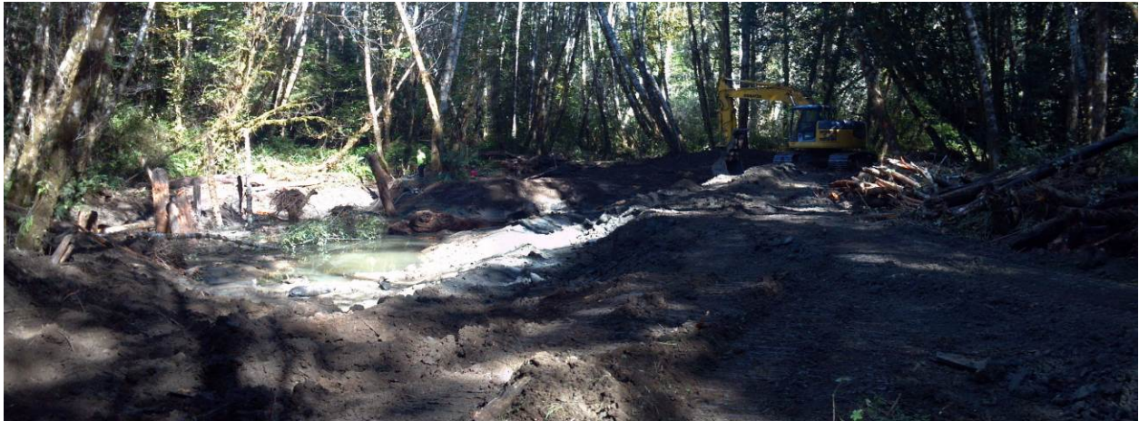
Photo-Site McGAlcoveIV_1: McGarvey Creek Alcove IV during construction (10/12/2014).
