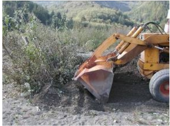
Figure 39. Construction of a willow siltation baffles in lower Terwer Creek, Lower Klamath River Sub-basin, California (2004) (Note the large wood placed at the base of the baffle).
