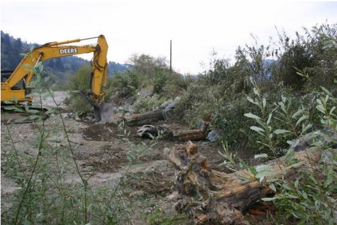
Figure 48. Construction of large wood-boulder structures in lower Terwer Creek, Lower Klamath River Sub-basin, California (2005).
