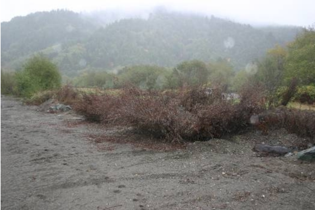
Figure 52. Newly constructed willow siltation baffles and mattresses along the east bank of lower Terwer Creek Lower Klamath River Sub-basin, California (2006).
