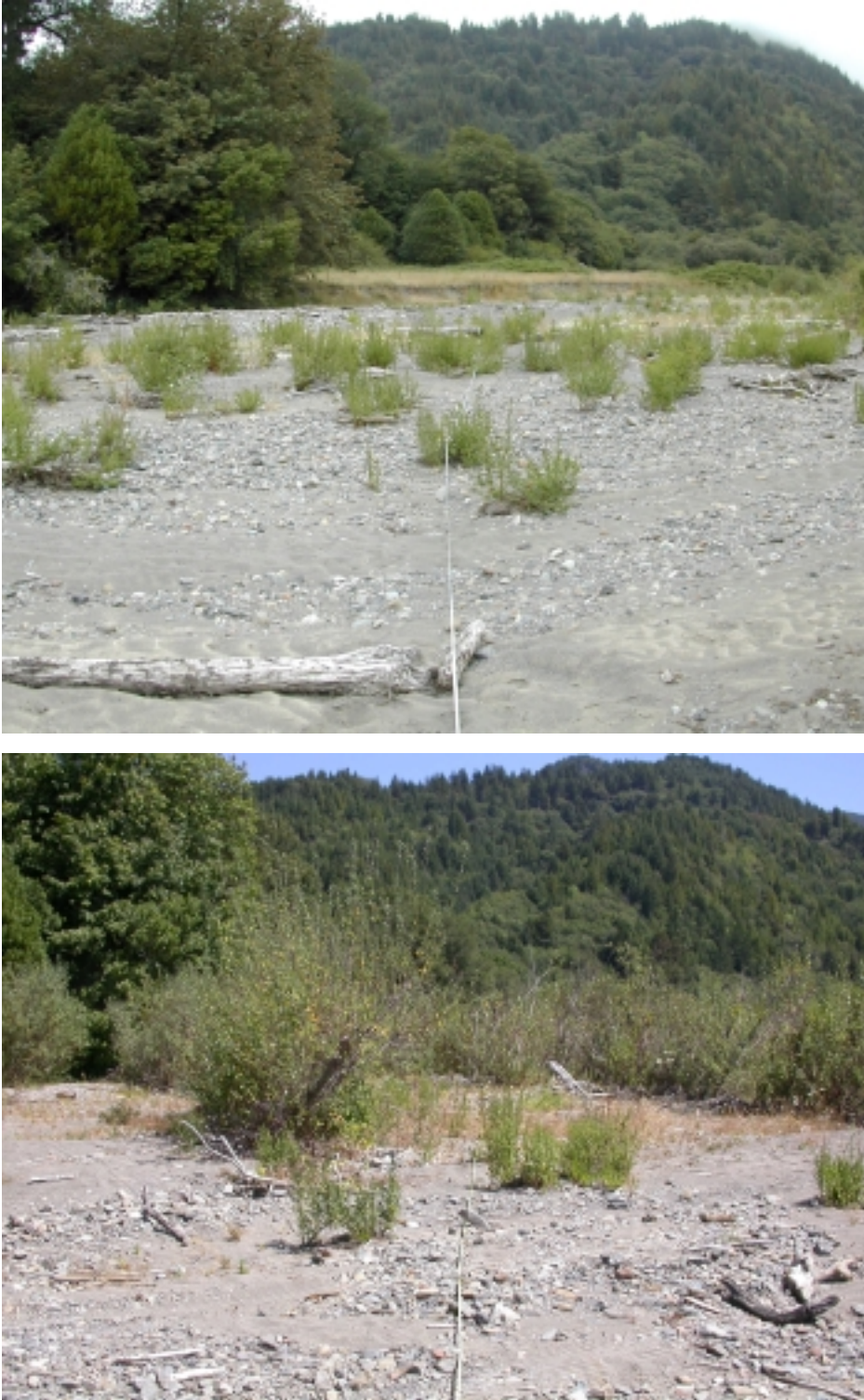
Figure 42. Photographs taken from a permanent photographic monitoring point in Terwer Creek, Lower Klamath River Sub-basin, California. The top photograph depicts pre-project conditions (2004), while the bottom photograph depicts newly constructed willow siltation baffles on the floodplain (2005).
