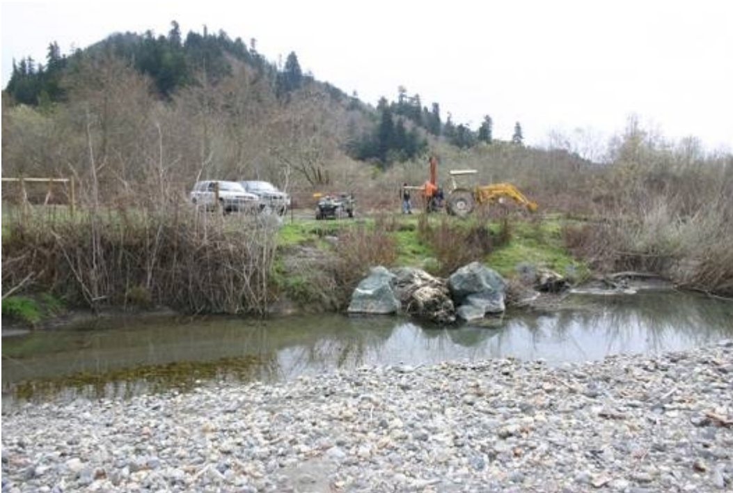
Figure 53. Large wood-boulder structure constructed along the east bank of lower Terwer Creek, Lower Klamath River Sub-basin, California (2008).
