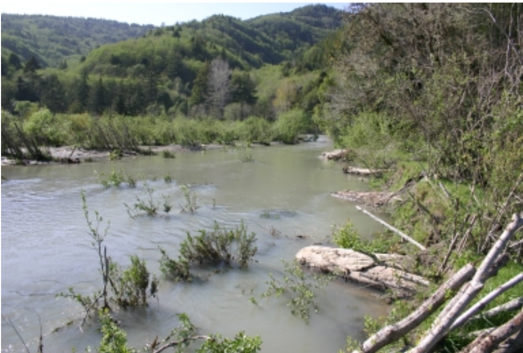
Figure 40. Large wood and willow structures following construction (top photograph 2005) and during a moderate flow event (bottom photograph 2005), lower Terwer Creek, Lower Klamath River Sub-basin, California.
