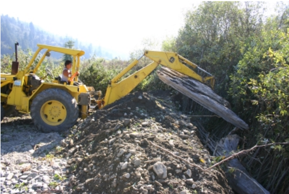
Figure 47. Placement of large wood at the base of a willow mattress constructed in lower Terwer Creek, Lower Klamath River Sub-basin, California (2005).
