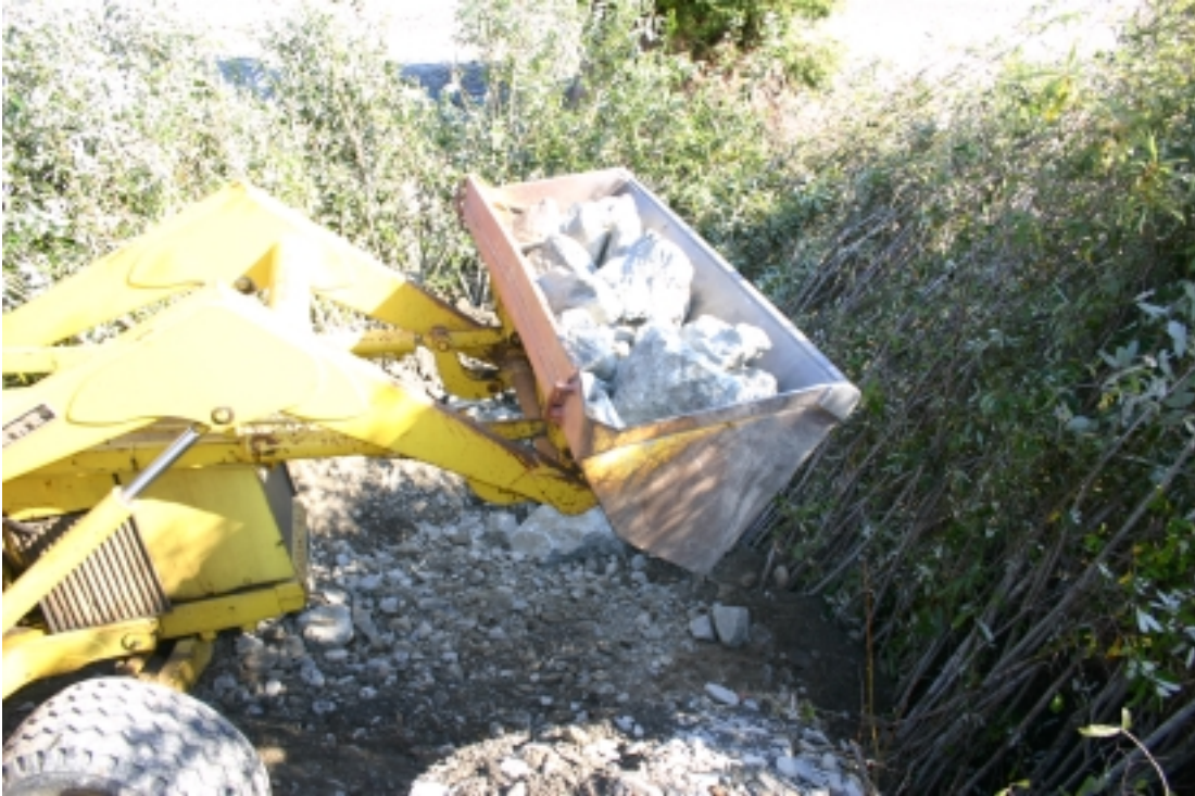
Figure 46. Placement of ¼ ton quarry rock at the base of a willow siltation baffle constructed in lower Terwer Creek, Lower Klamath River Sub-basin, California (2005).
