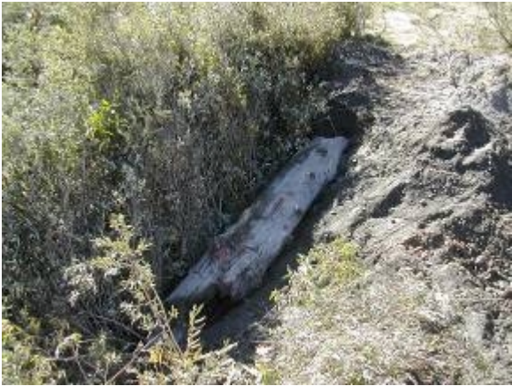
Figure 39. Construction of a willow siltation baffles in lower Terwer Creek, Lower Klamath River Sub-basin, California (2004) (Note the large wood placed at the base of the baffle).
