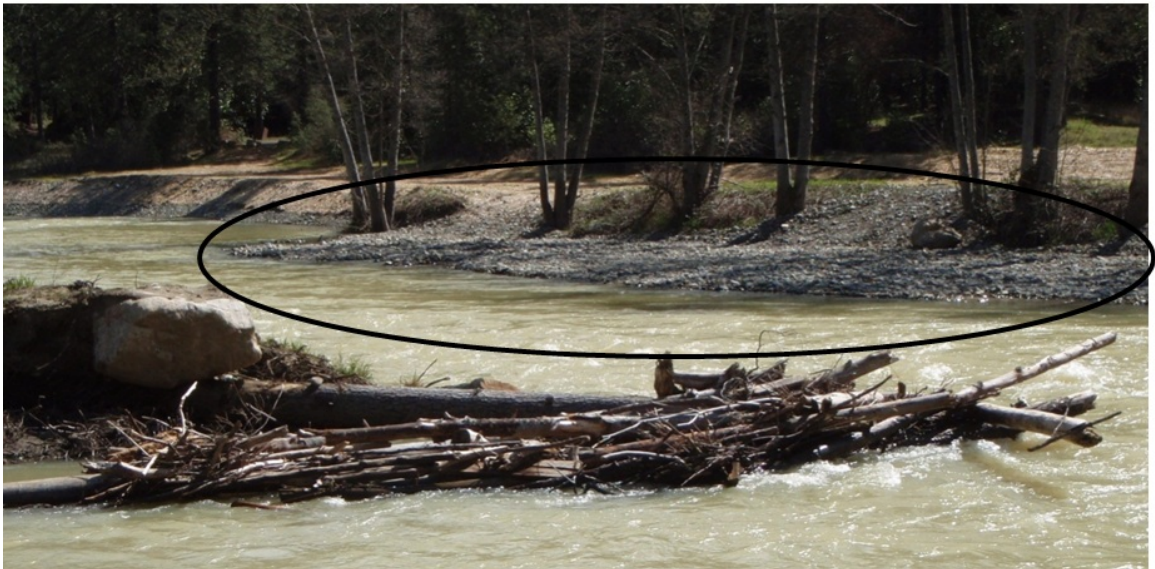
Figure 21. Post-construction (pre-high-flow) photos of the IC-2 constructed point bar at Lowden Meadows rehabilitation site (upper photo) and the IC-7 constructed point bar (pre-high flow) at Reading Creek rehabilitation site (lower photo). Discharges at the Lowden Meadows site were 14.3 cms (506 cfs) and were 31.1 cms (1,100 cfs) at the Reading Creek site during the time the photos were taken.
