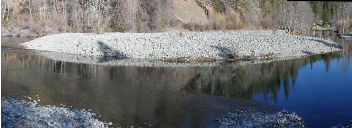
Figure 22. Post-2011 high flow photo of the IC-2 constructed point bar at Lowden Meadows.
