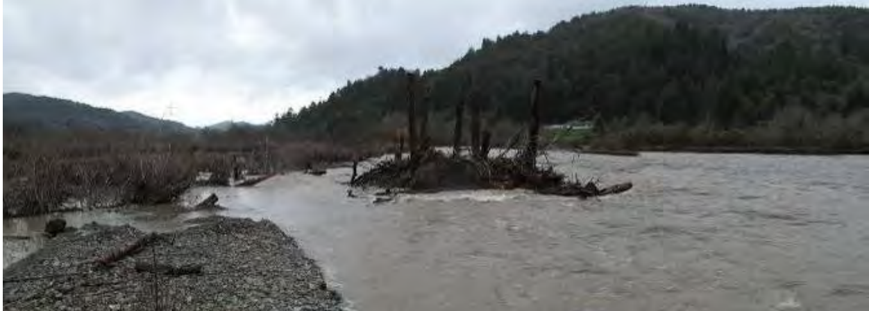
Figure 2. Looking downstream at Terwer ELJ 1 and willow baffles protecting a side channel and Holocene soils and creating low velocity habitat (01/01/10 - near bankfull event ~1,600 cfs).
