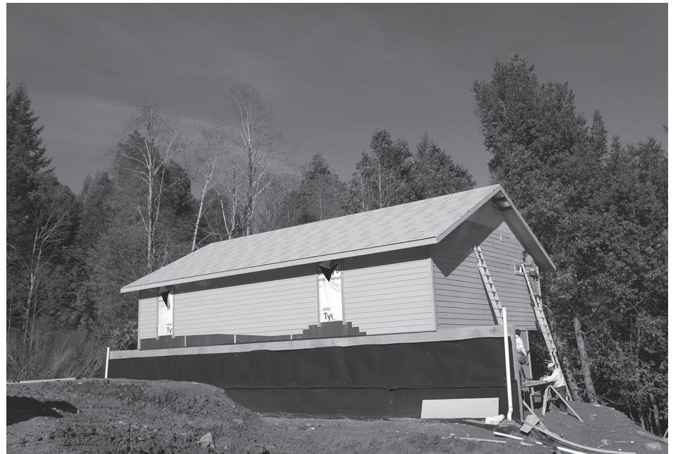
Here is the first-ever upriver police station.
