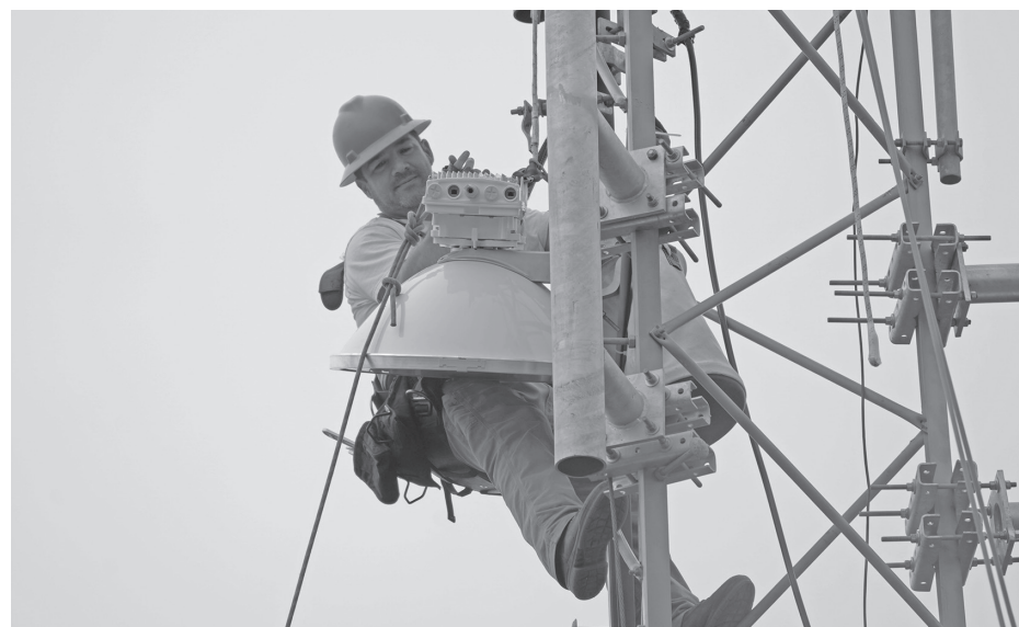
Yurok Connect Coordinator Duston Offins installs new equipment.
