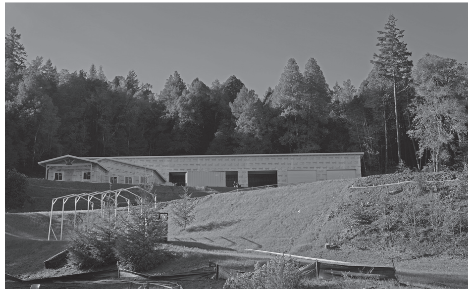
This 10,946 square-foot building will be shared by the Yurok Fire Department and Yurok OES.
