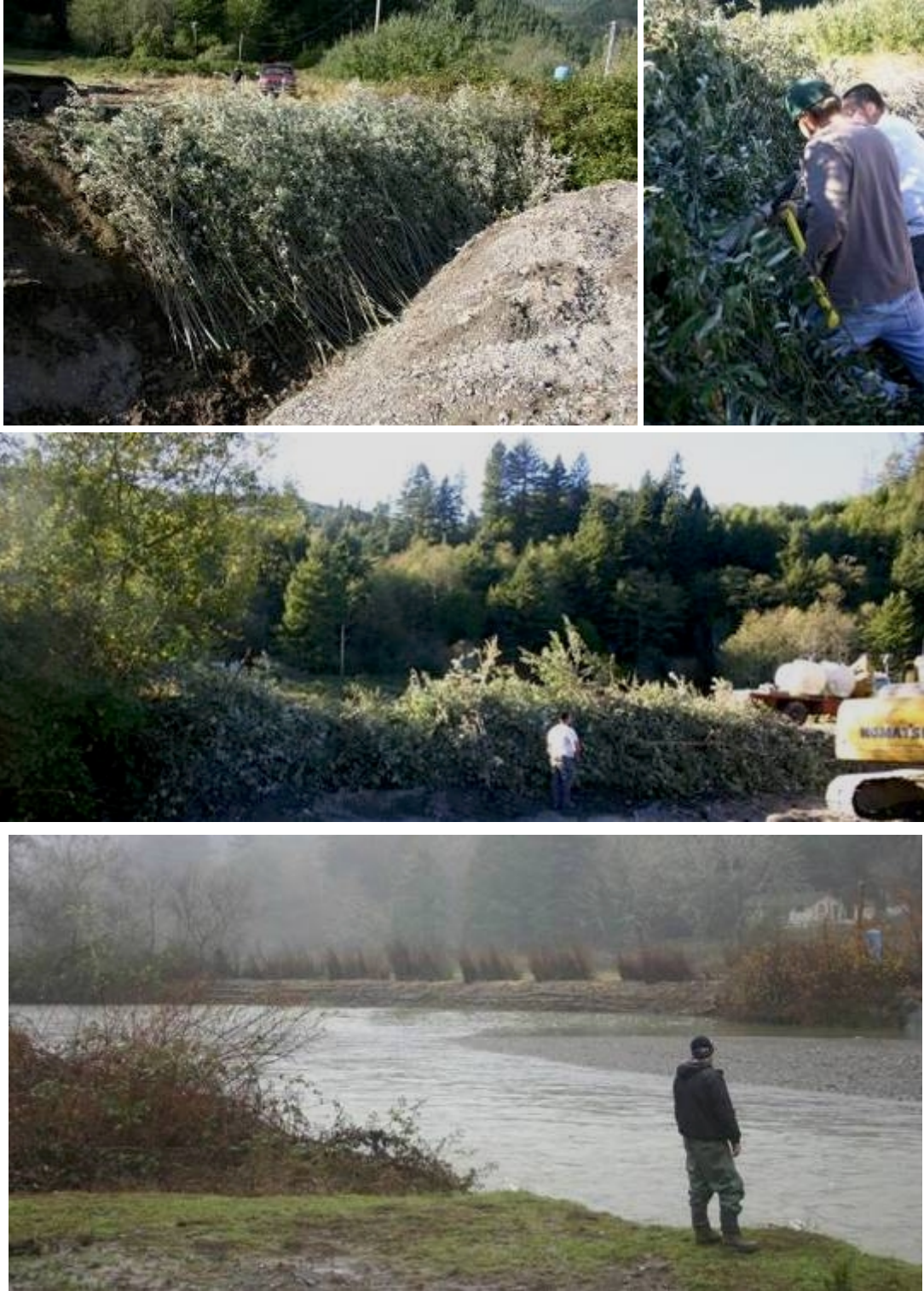
Figure 10. Yurok Tribal Fisheries Program staff working with a local landowner to construct a willow mattress in lower Terwer Creek (Top and Middle - October 2008); and the constructed willow mattress and baffles during winter flows (Bottom - January 2009).
