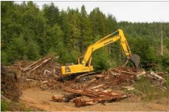
Figure 3. Yurok Tribal Fisheries Program and Fiori GeoSciences transforming slash piles and whole tree materials into fish habitat in the McGarvey Creek watershed (2009).
