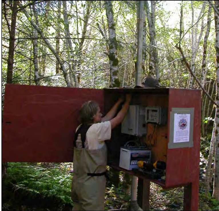
Figure 27. Tully Creek gage station condition pre-flood (October 2004).
