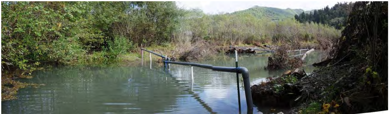
Figure 21. Photographs of the outlet channel of Terwer Creek Pond A (Top) the PIT tag antenna arrays (Top and Bottom), and of the habitat structures constructed in the pond (Bottom).
