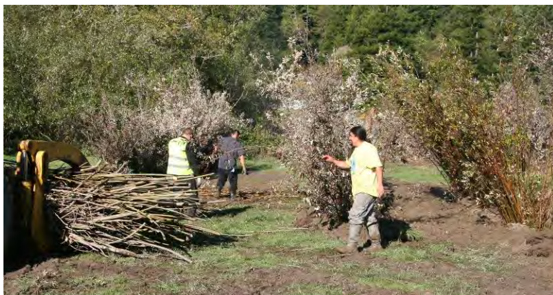
Figure 13. Photographs of willow baffle construction in Lower Terwer Creek using LWD.
