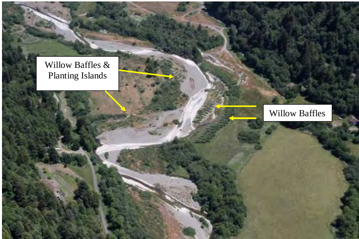
Figure 10. Aerial photograph of lower Terwer Creek depicting recently constructed willow baffles and planting islands, Lower Klamath River (Summer 2011).
