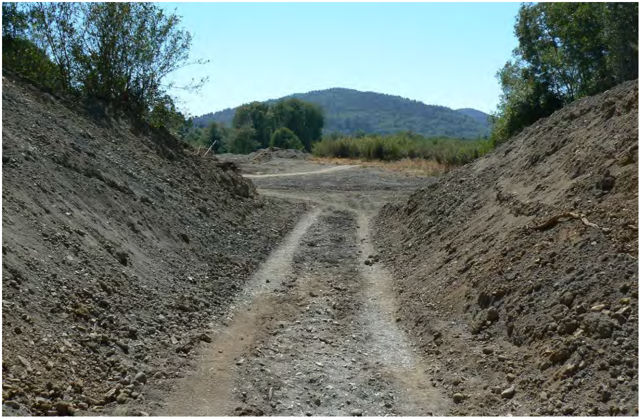
Figure 25. Photographs looking upstream at the breached levee and existing wetland habitats (Top) and looking downstream through the breached levee during off-channel habitat enhancement of Terwer Creek Pond B, Lower Klamath River (summer 2010).
