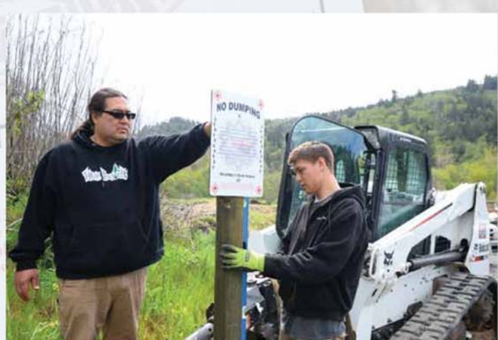
(Left) Roger Boulby and his son Robert helped YTEP install "No Dumping" signs as part of the 18th Annual Klamath River Clean Up
