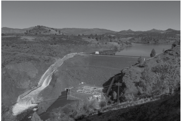
Iron Gate is the first of four dams slated for decommissioning in 2021.
