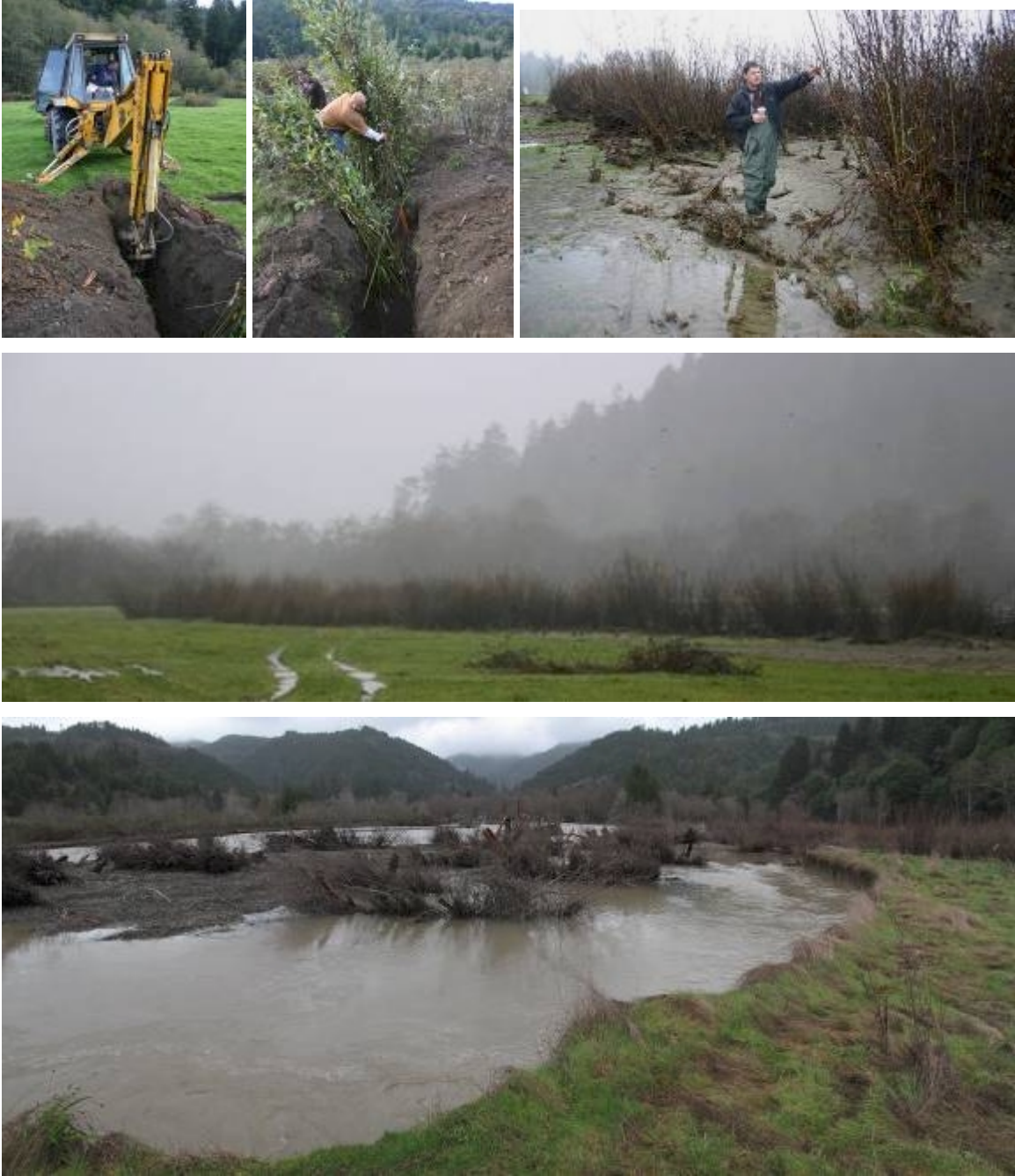
Figure 6. Photographs of willow baffle construction (Top Left – winter 2009) and following construction and high flow events (Top Right and Middle and Bottom).
