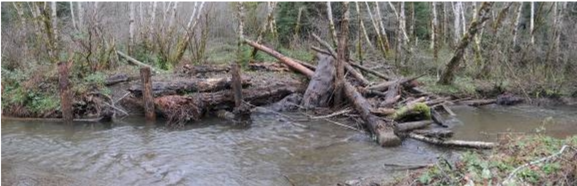
Figure 2. Photographs of the 2009 Site 5 prior to wood loading activities (Top – Summer 2009) and following construction of the wood jam (Bottom – Fall 2009).
