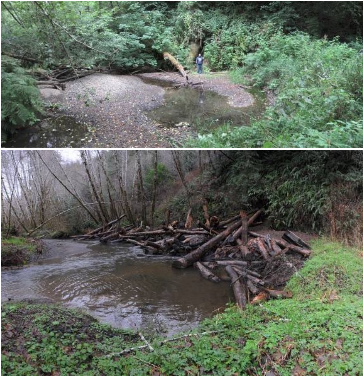
Figure 1. Photographs of the 2009 Site 5 prior to wood loading activities (Top – Summer 2009) and following construction of the wood jam (Bottom – Fall 2009).
