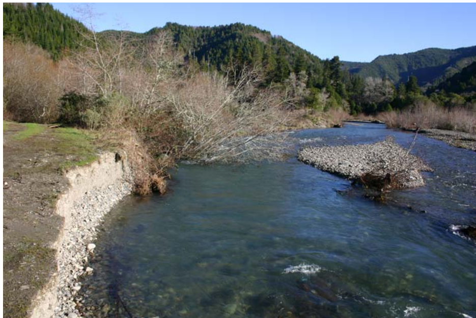
Figure 7. Streambank erosion at upper half of project site, Lower Terwer Creek , Lower Klamath River, California, January 24, 2006.
