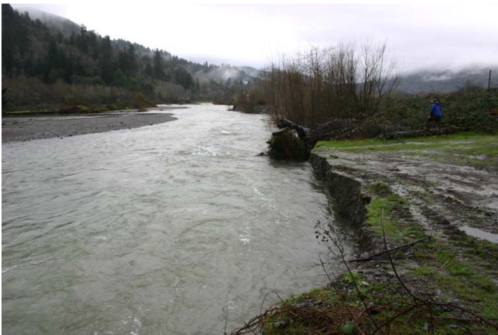
Figure 5. Streambank erosion at lower half of project site, Lower Terwer Creek , Lower Klamath River, California, January 20, 2006.
