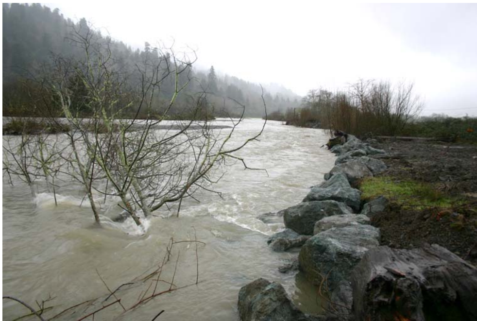
Figure 13. Stabilized streambank viewed from upper end of project site, Lower Terwer Creek ,Lower Klamath River, California, February 01, 2006.
