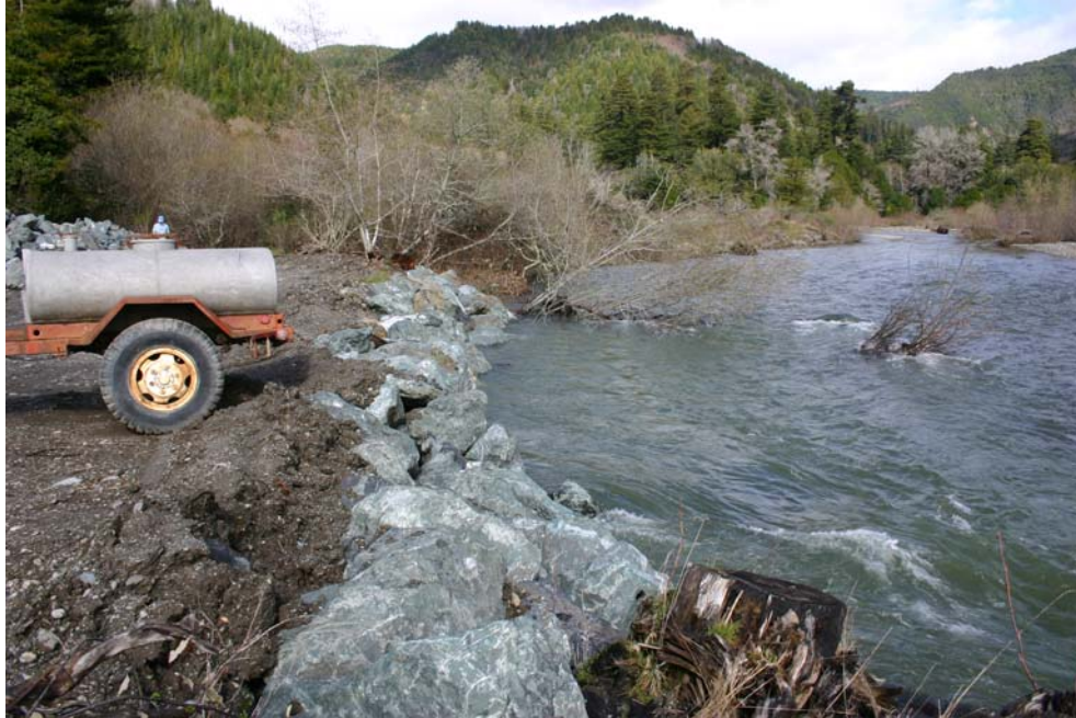
Figure 14. Stabilized streambank viewed from lower end of project site, Lower Terwer Creek, Lower Klamath River, California, February 28, 2006.
