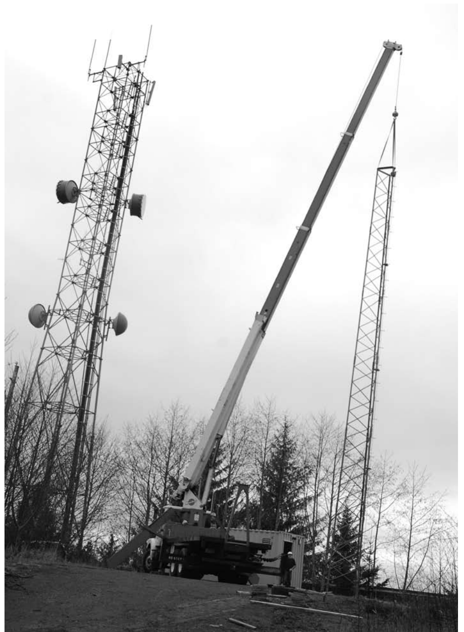
A new wireless tower is erected on Requa Hill.
