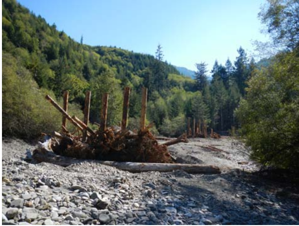
Figure 6. Large bar apex jams constructed in Terwer Creek Gage Reach (October 2015).
