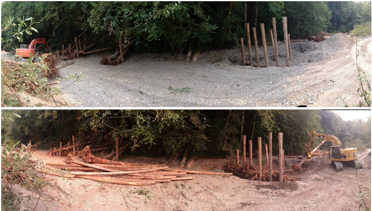
Figure 5. Constructed wood jams in Hunter Creek during installation (October 2015).
