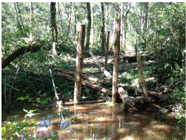
Figure 8. A constructed wood jam in Waukell Creek during installation (Left) and as-built (Right - September 2015).
