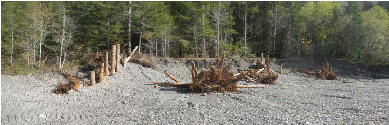
Figure 7. A series of constructed wood jams along a stream bank in Terwer Creek Gage Reach.
