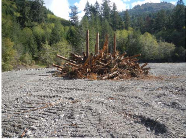
Figure 6. Large bar apex jams constructed in Terwer Creek Gage Reach (October 2015).
