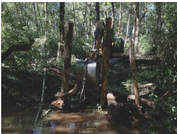
Figure 8. A constructed wood jam in Waukell Creek during installation (Left) and as-built (Right - September 2015).
