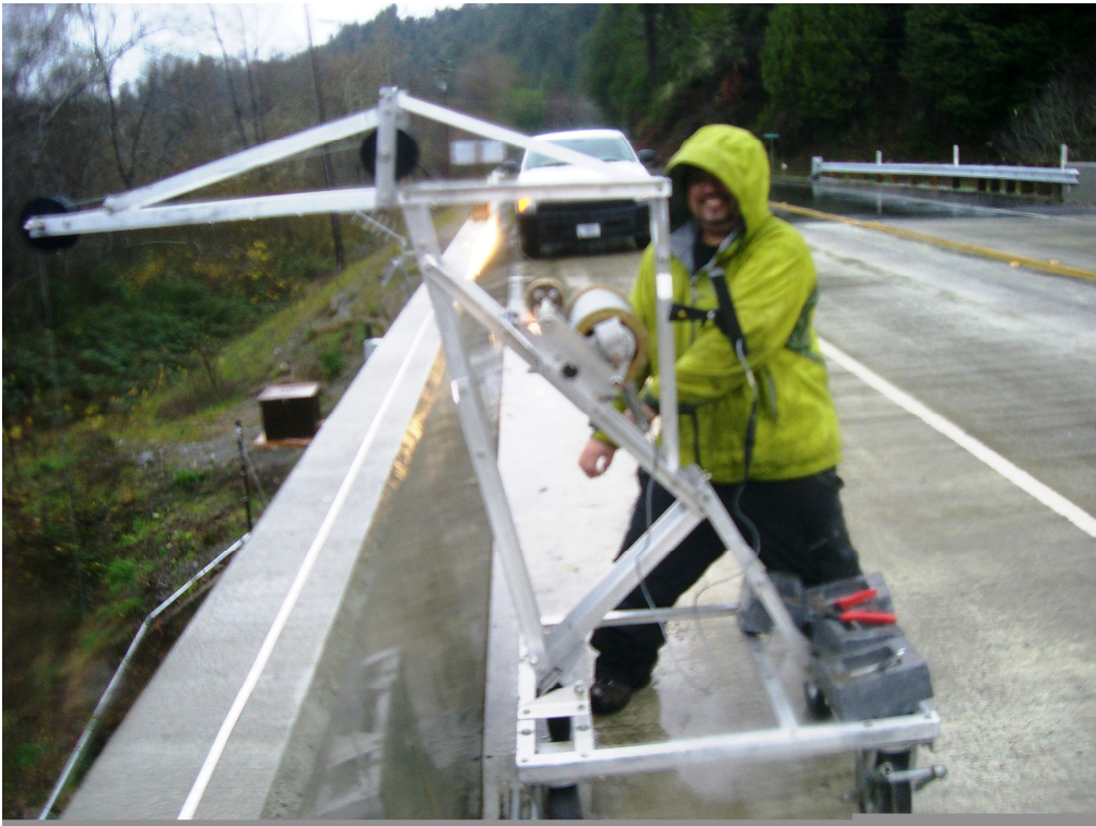
Figure 8. Photo of Micah Gibson operating the bridge crane, Lower Turwar Creek, December 27, 2007.
