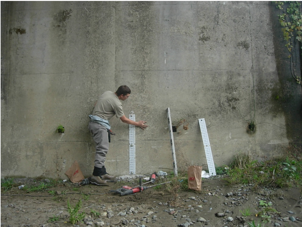
Figure 6. Photo of Ken Fetcho mounting staff plate on bridge abutment Lower Turwar Creek, WY 2008.
