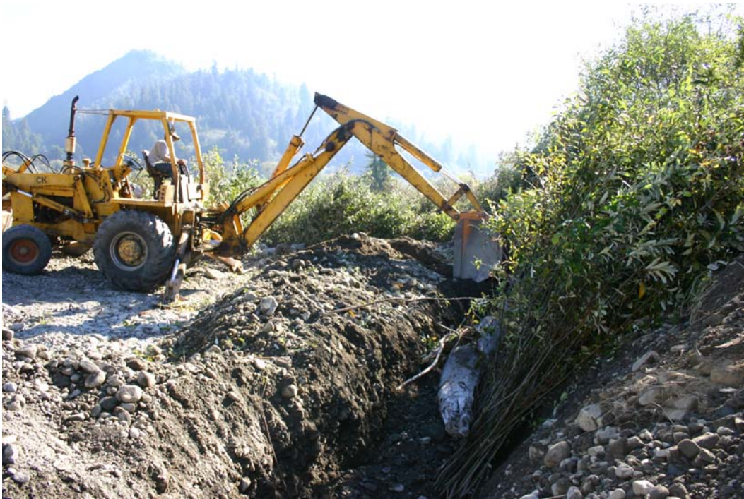
Figure 14. Backfilling willow mattress trench, Lower Terwer Creek, Lower Klamath River California, 2005.
