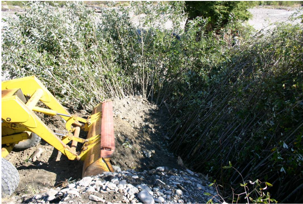
Figure 11. Backfilling willow siltation baffle, Lower Terwer Creek, Lower Klamath River California, 2005.
