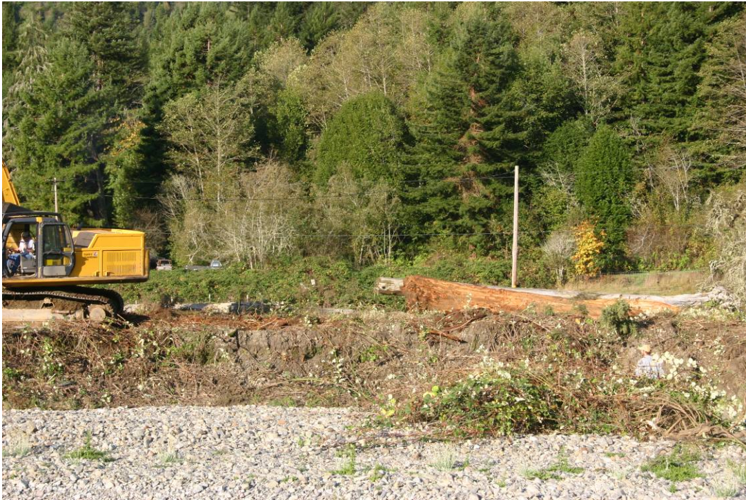
Figure 19. Removing non-native blackberries from highly erosive streambank, Lower Terwer Creek, Lower Klamath River California, 2005.
