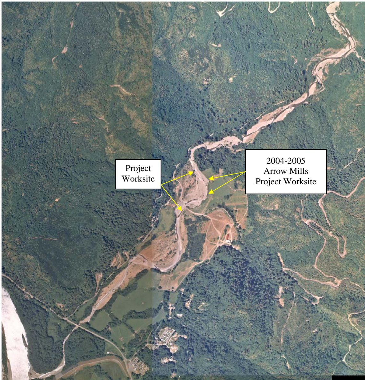
Figure 2. Aerial view of the lower 3.0 miles of Terwer Creek, Lower Klamath River, California, 1997.
