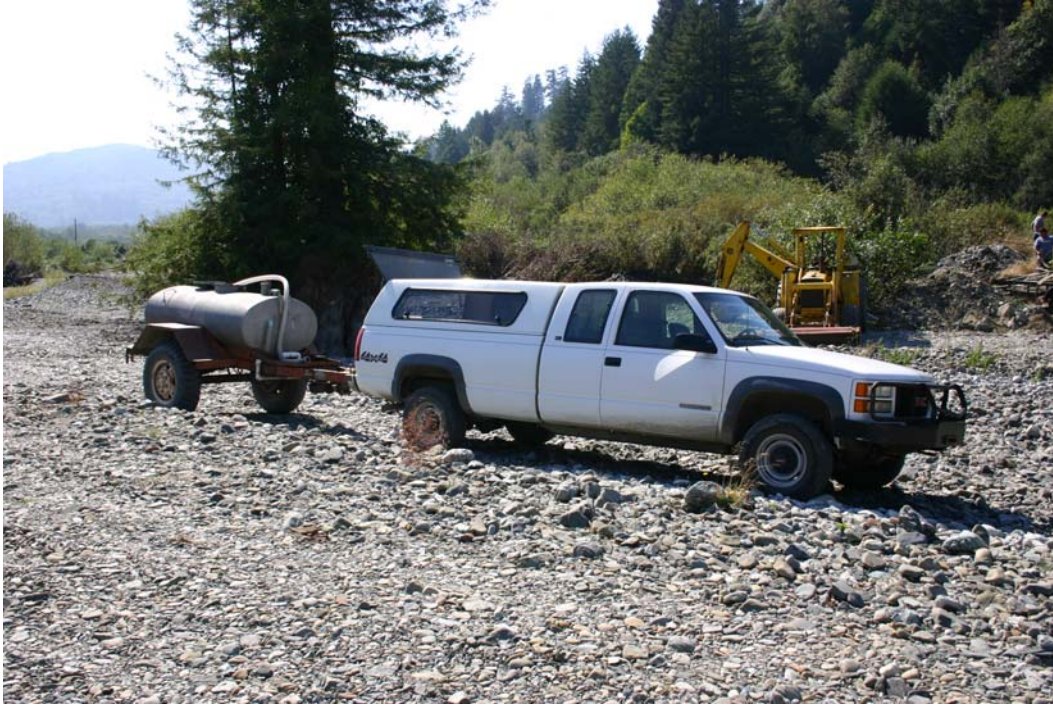
Figure 15. Delivering water to willow siltation baffle installation site, Lower Terwer Creek, Lower Klamath River, California, 2005.
