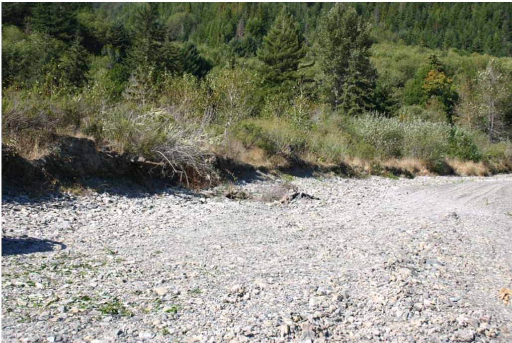
Figure 6. Upper end of willow baffle/mattress project site before construction, Lower Terwer Creek, Lower Klamath River, California, 2005.
