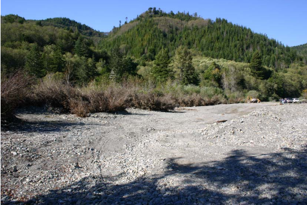
Figure 17. Project site following installation of willow baffles/mattresses, Lower Terwer Creek, Lower Klamath River, California, 2005.
