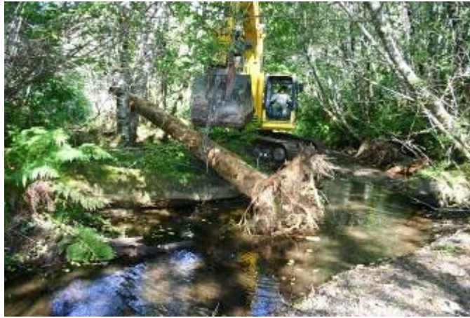
b. Using an excavator to wedge large wood into existing vegetation.
