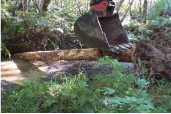
a. Using an excavator to insert large wood into the bank.
