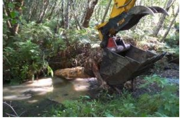
a. Using an excavator to insert large wood into the bank.
