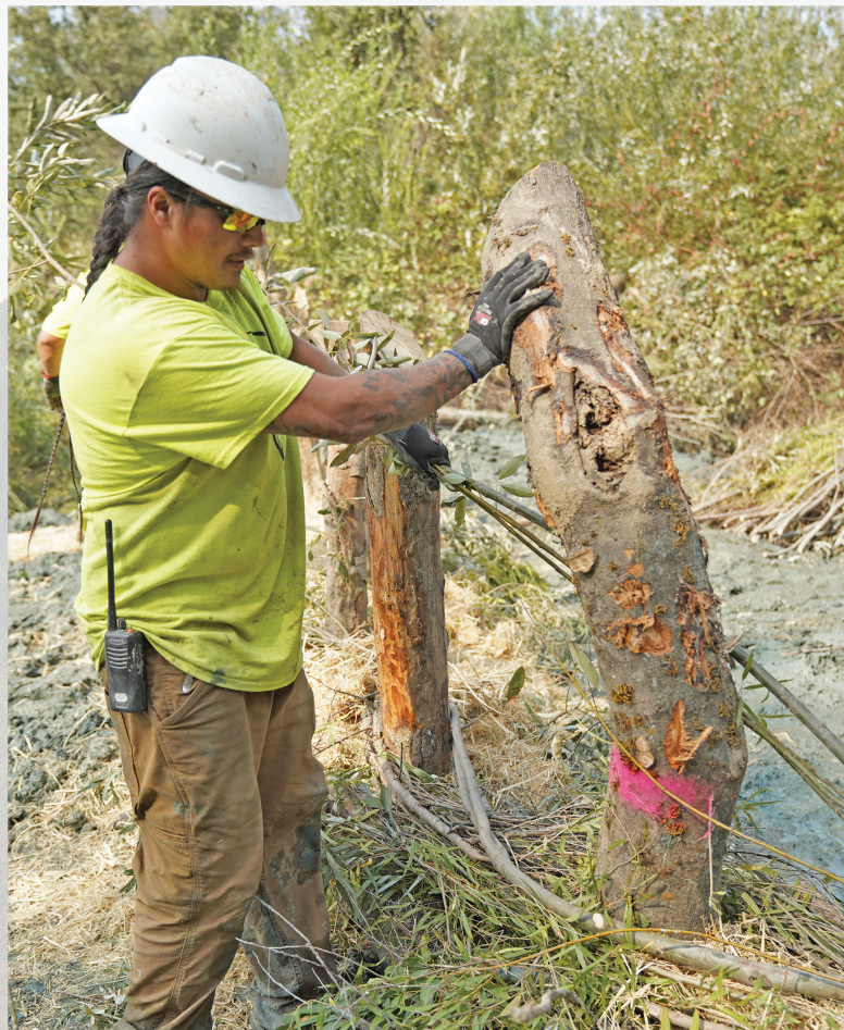
The Yurok Fisheries Department's Richard Bates II helps construct a beaver dam analogue.
