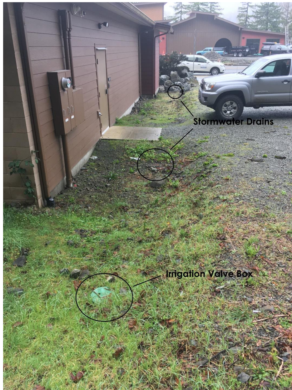
Figure 6 South wall of existing structure showing irrigation valve box, stormwater drains, and various utilities on the north wall of the existing structure (looking west)
