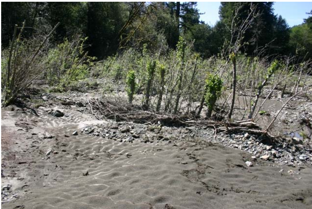
Figure 31. Willow baffles at lower end of site showing new growth, Lower Terwer Creek, Lower Klamath River, California, 2005.
