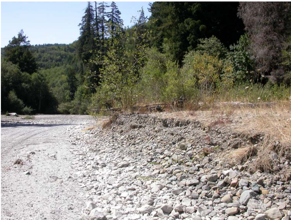
Figure 35. Photographs taken from a permanent photographic monitoring point in Terwer Creek, Lower Klamath River. The upper photograph was taken in summer 2004 and the lower photograph was taken in summer 2005. Note the newly eroded stream bank in the 2005 photograph.
