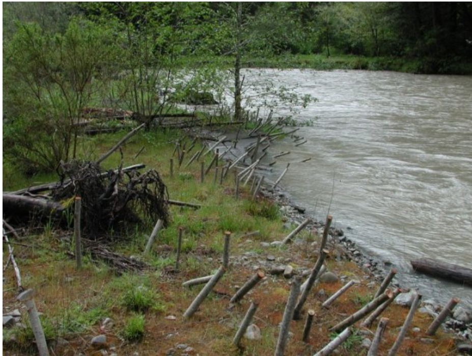
Figure 21. Willow posts installed along streambank, Lower Terwer Creek, Lower Klamath River, California, 2004.
