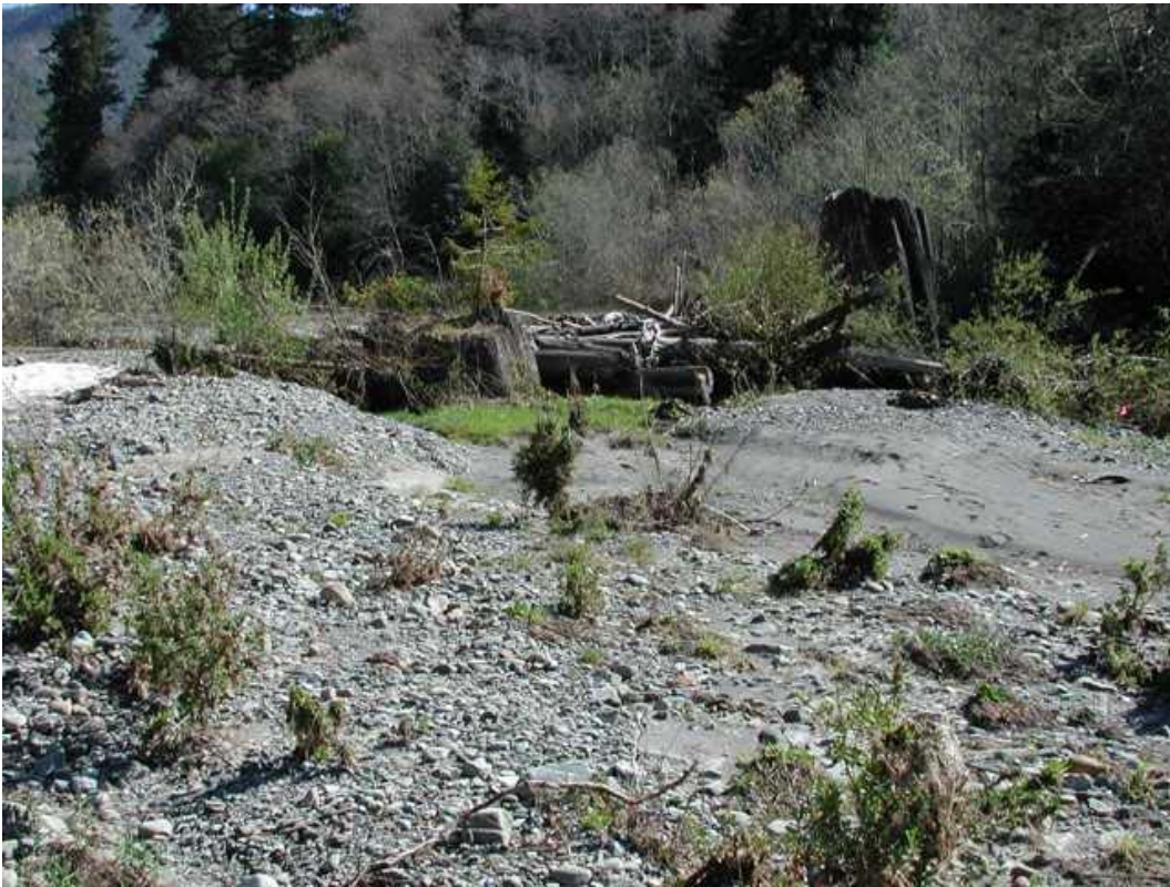
Figure 26. Upper end of willow baffle/mattress project site before construction, Lower Terwer Creek, Lower Klamath River, California, 2004.
