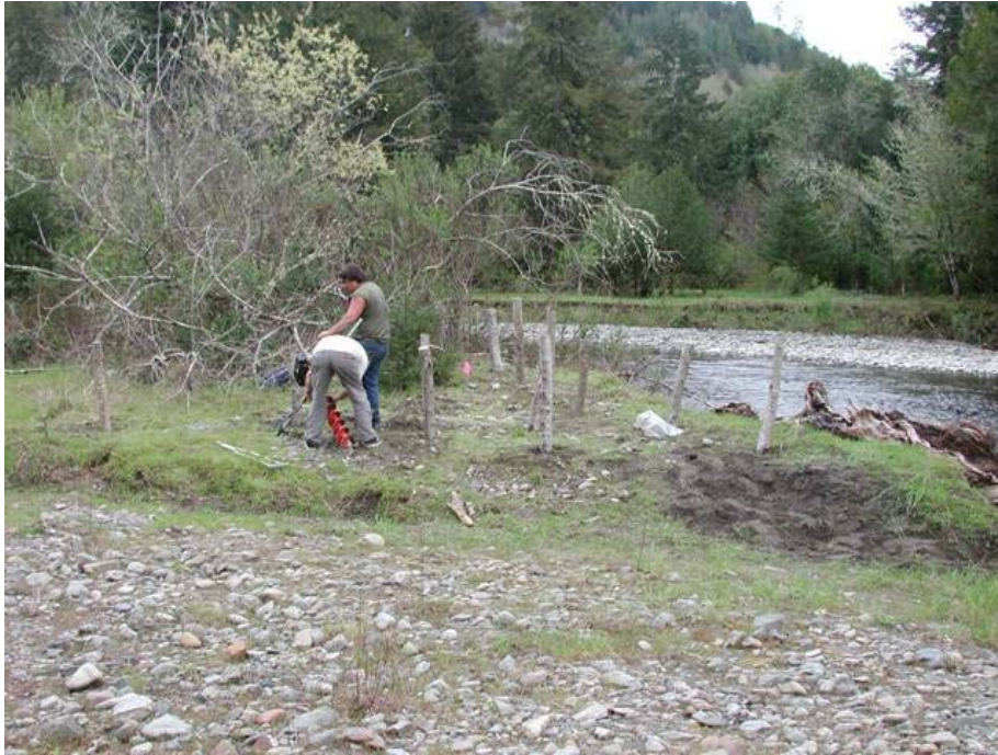
Figure 20. YTFP crew installing willow posts, Lower Terwer Creek, Lower Klamath River, California, 2004.
