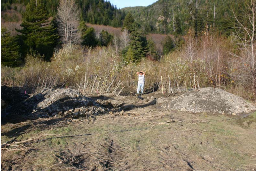
Figure 50. YTFP staff installing willow baffles on adjoining flood terrace, Lower Terwer Creek, Lower Klamath River, 2005.
