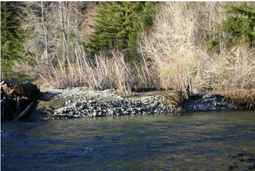
Figure 27. Willow baffles at upper end of site after installation, Lower Terwer Creek, Lower Klamath River, California, 2005
