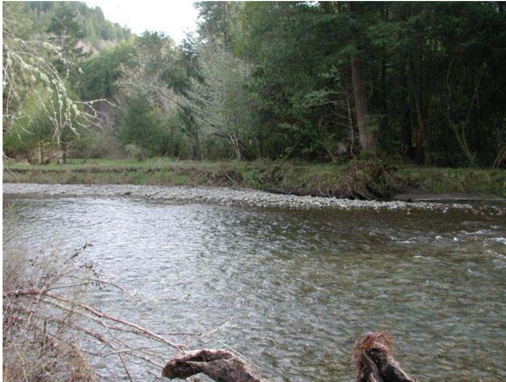
Figure 22. Eroding streambank on east side of creek, Lower Terwer Creek, Lower Klamath River, California, 2004.
