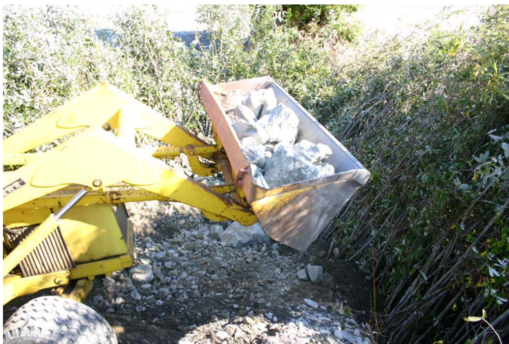
Figure 43. Placing quarter-ton quarry rock on willow siltation baffle, Lower Terwer Creek, Lower Klamath River, California, 2005.
