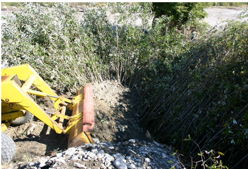
Figure 42. Backfilling willow siltation baffle, Lower Terwer Creek, Lower Klamath River California, 2005.
