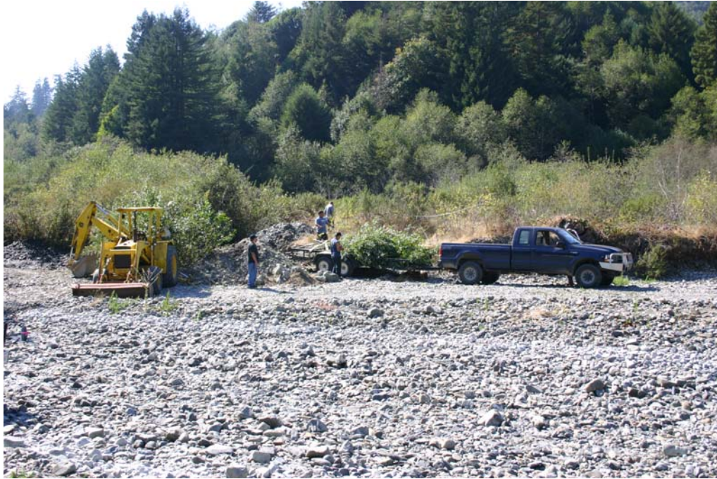
Figure 40. YTFP staff constructing willow siltation baffle, Lower Terwer Creek, Lower Klamath River California, 2005.
