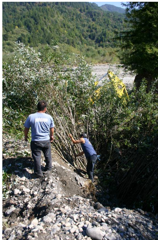
Figure 41. YTFP staff constructing willow siltation baffle, Lower Terwer Creek, Lower Klamath River California, 2005.
