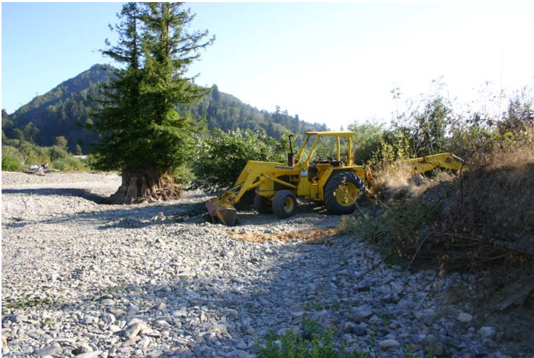
Figure 39. Excavating willow siltation baffle trench at lower end of baffle/mattress project site, Lower Terwer Creek, Lower Klamath River, California, 2005.
