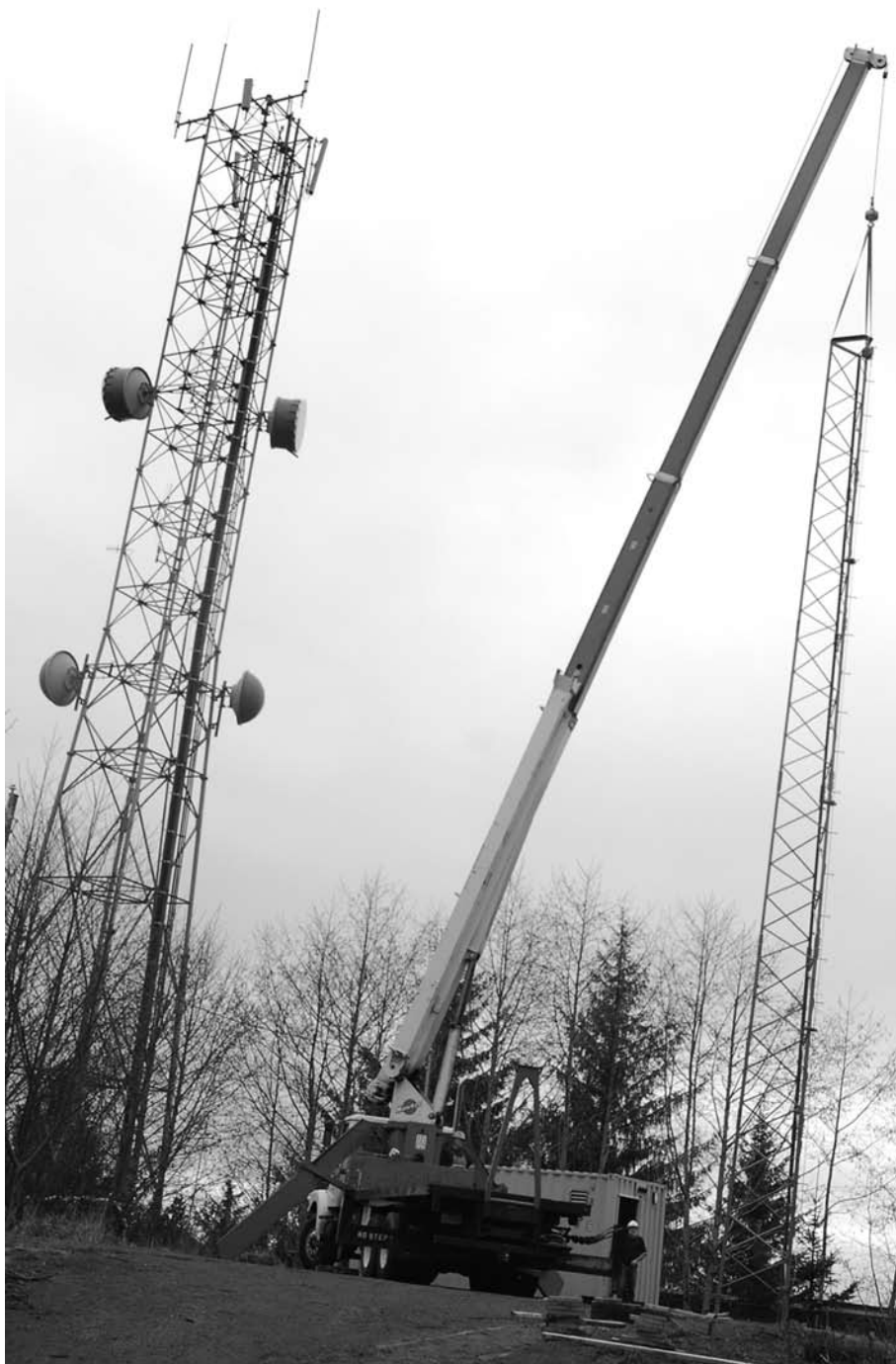
The first tower is set up on Requa Hill.
