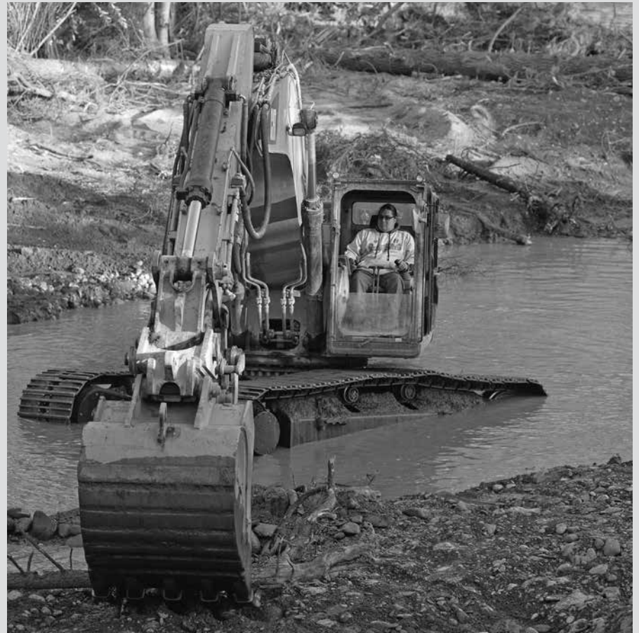
Yurok Tribal member Roger Boulby works on the Bucktail Project.
